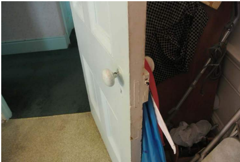
Plate 30: Detail of hardware located on a first-floor door.
