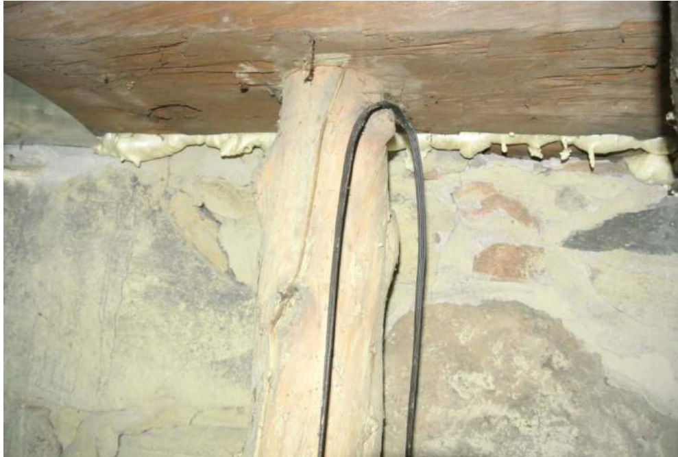
Plate 55: Detail of log support posts and hewn beams.
