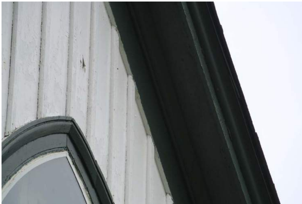
Plate 8: Detail of board-and-batten cladding and wood soffit and fascia.
