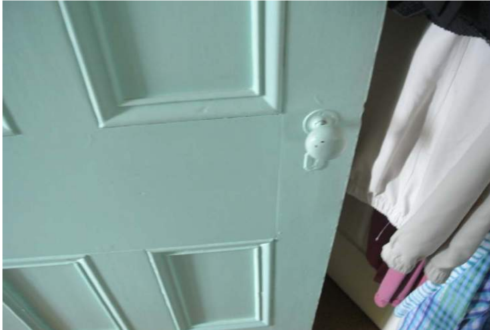
Plate 43: Detail of original hardware.
