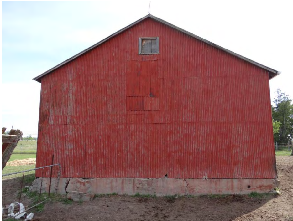
Plate 100: West elevation of drive shed one (D1).
