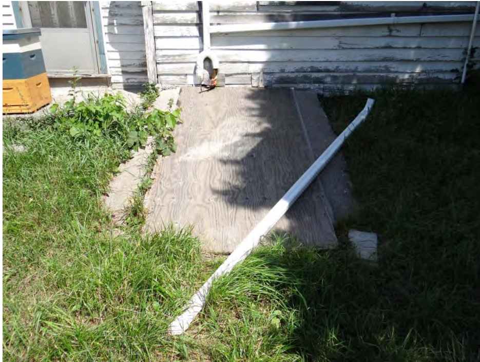
Plate 23: Photo of the storm door located on the south elevation.
