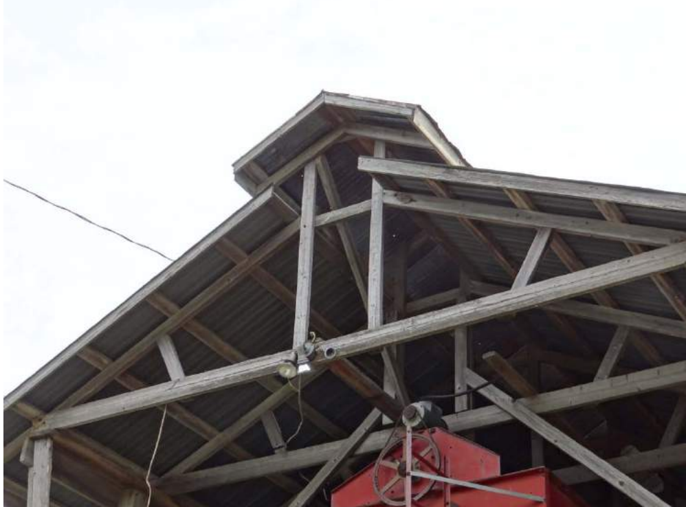
Plate 64: Detail of the monitored roof of Outbuilding 1.
