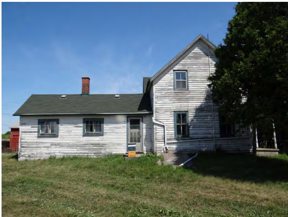
Plate 2: South elevation of the farmhouse.
