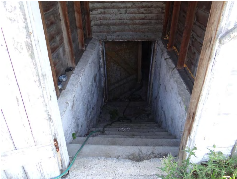
Plate 22: Interior door leading to the basement, west elevation.
