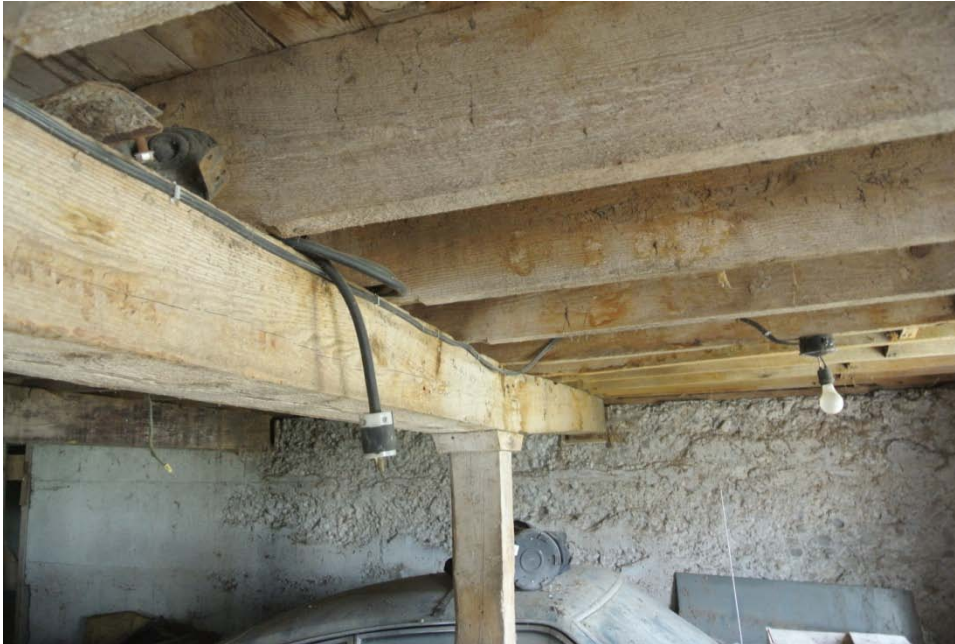
Plate 57: Detail of framing in lower level of the barn.
