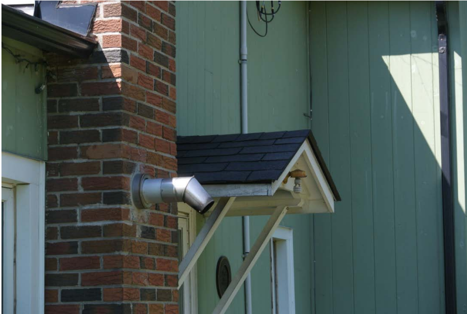
Plate 13: Cantilever porch overhang at rear entrance on the north elevation.
