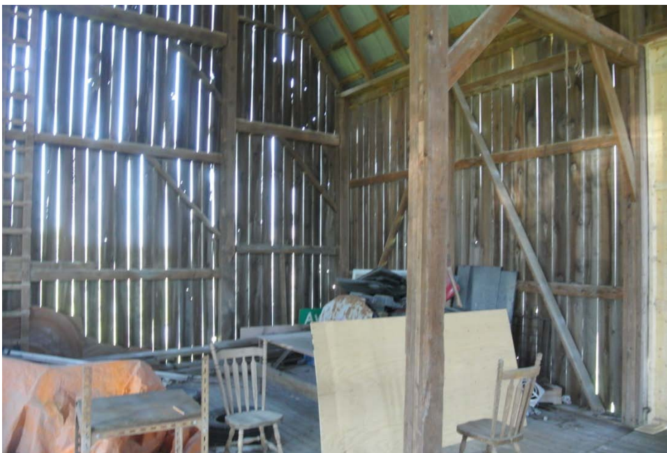
Plate 60: Detail of upper floor interior.
