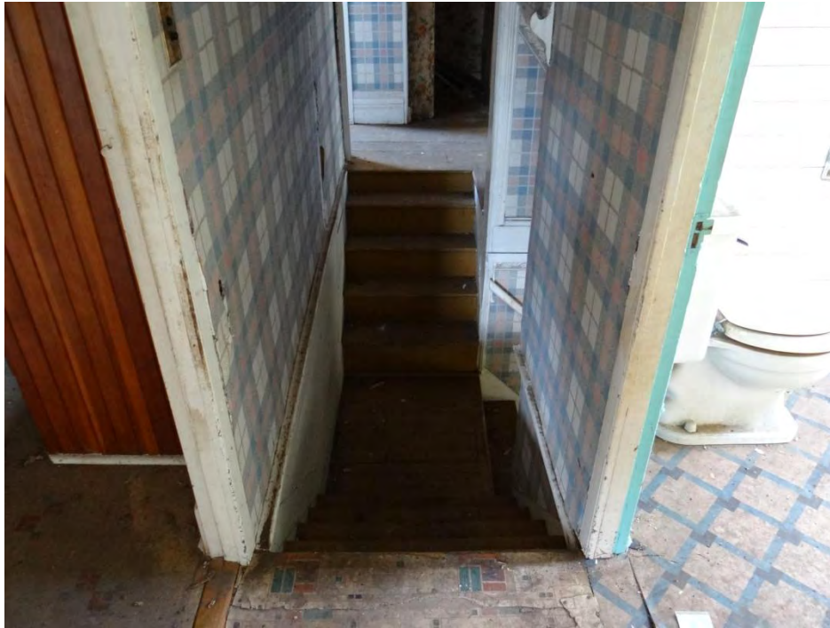
Plate 57: Photo of the landing at the top of the narrow stair case. The landing leads to two other sets of stairs, which lead to the bedroom one (master bedroom) and bedrooms two and three, respectively. Note the washroom in the foreground on the right.
