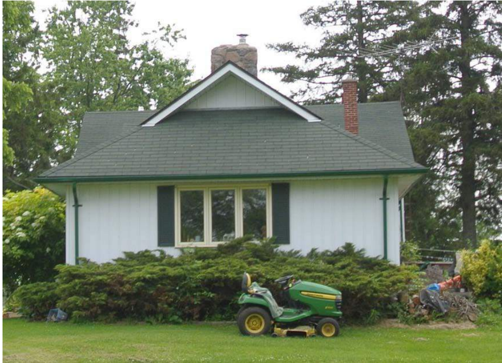
Plate 19: View toward the south elevation of the residence.
