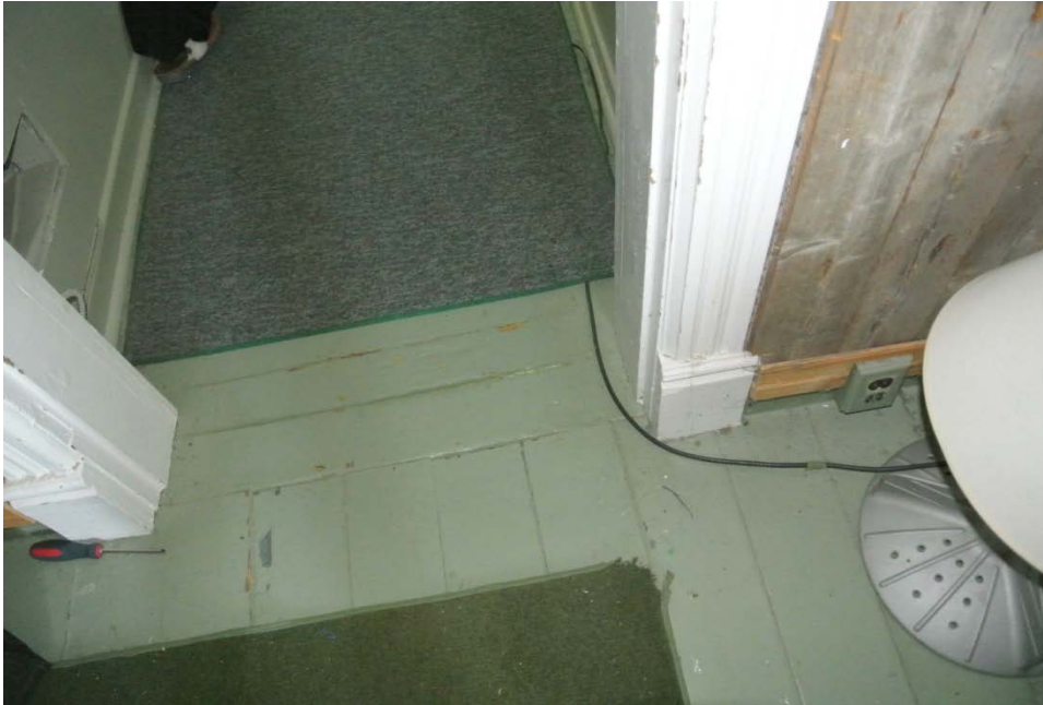
Plate 35: Detail of wood floor boards and door casing, upstairs landing.
