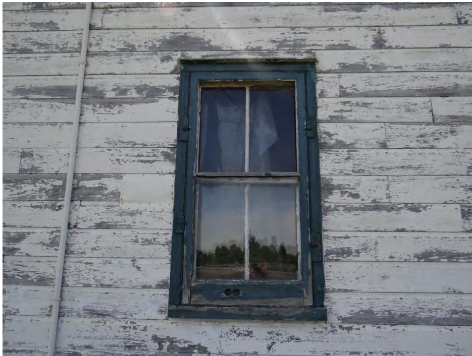
Plate 24: Two-over-two sash window located on the first storey of the original north section of the house (north elevation). Note the original storm cover.
