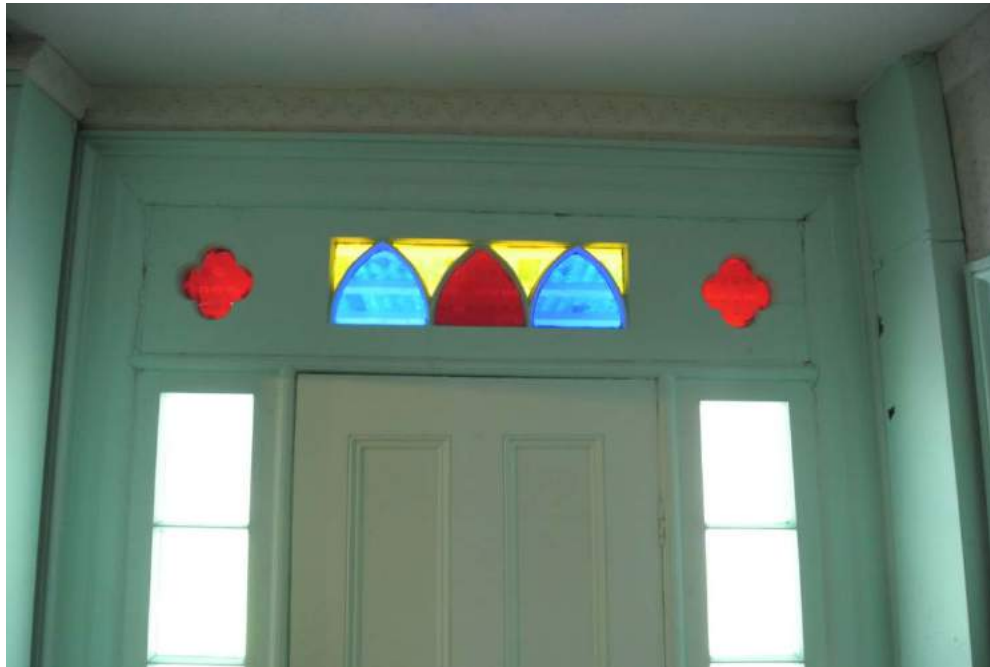
Plate 25: Detail of the transom and lights surrounding the central entryway.
