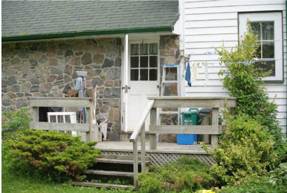
Plate 17: View toward the entry into the modern addition.
