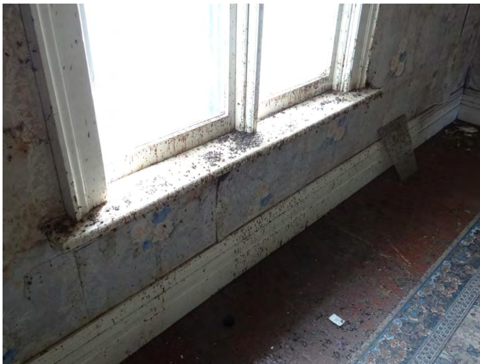
Plate 69: Photo of the moulded window sill and baseboard in bedroom two.
