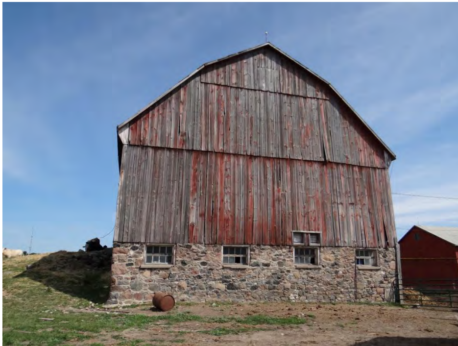
Plate 93: South elevation of the barn.
