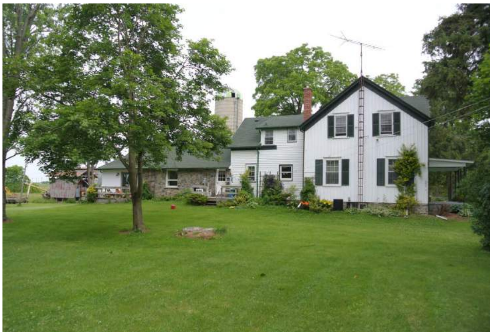
Plate 2: South elevation of residence.
