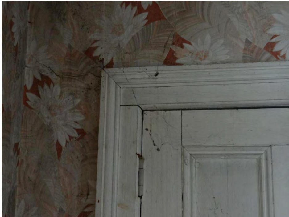
Plate 45: Detail of moulded door trim in living room two.
