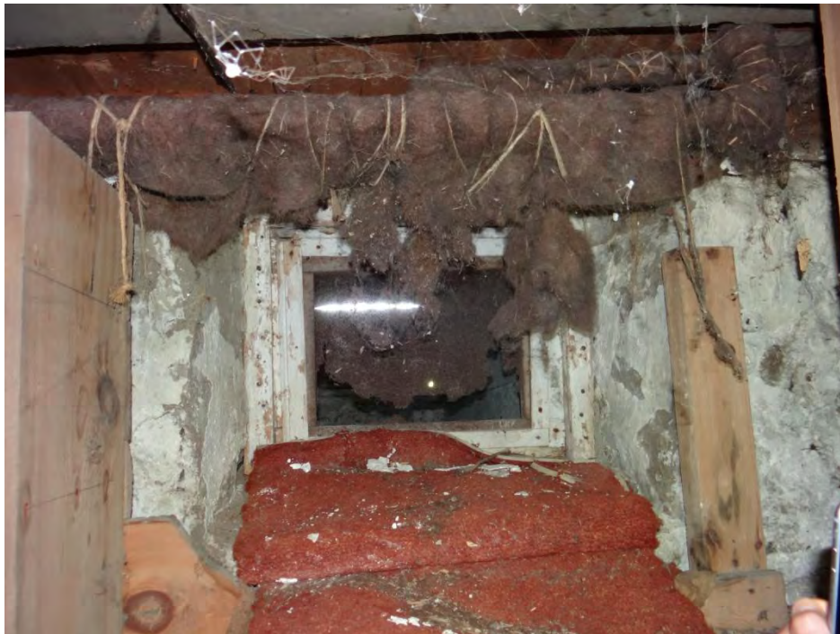
Plate 87: Photo of an exterior window in the basement (original south section).
