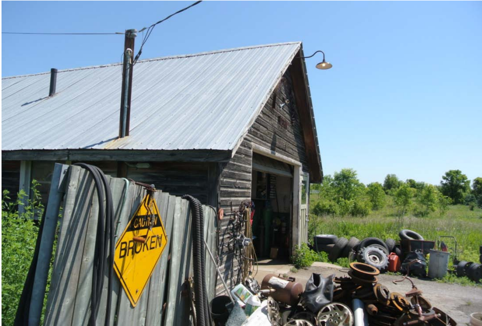
Plate 61: South and west elevation of the workshop.
