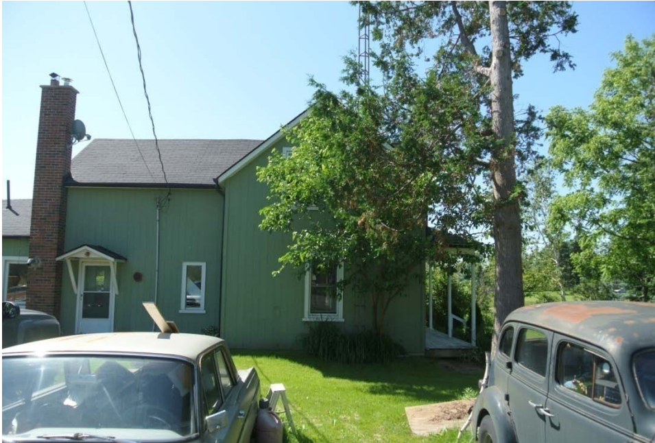
Plate 5: North elevation, detail of front part of the house.
