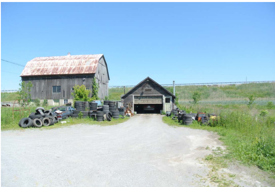
Plate 50: View of the two outbuildings located north of the farmhouse.
