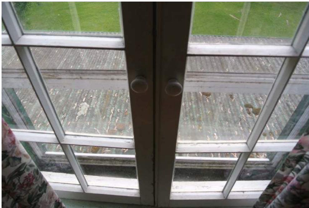
Plate 40: Detail of the centrally located arched window.
