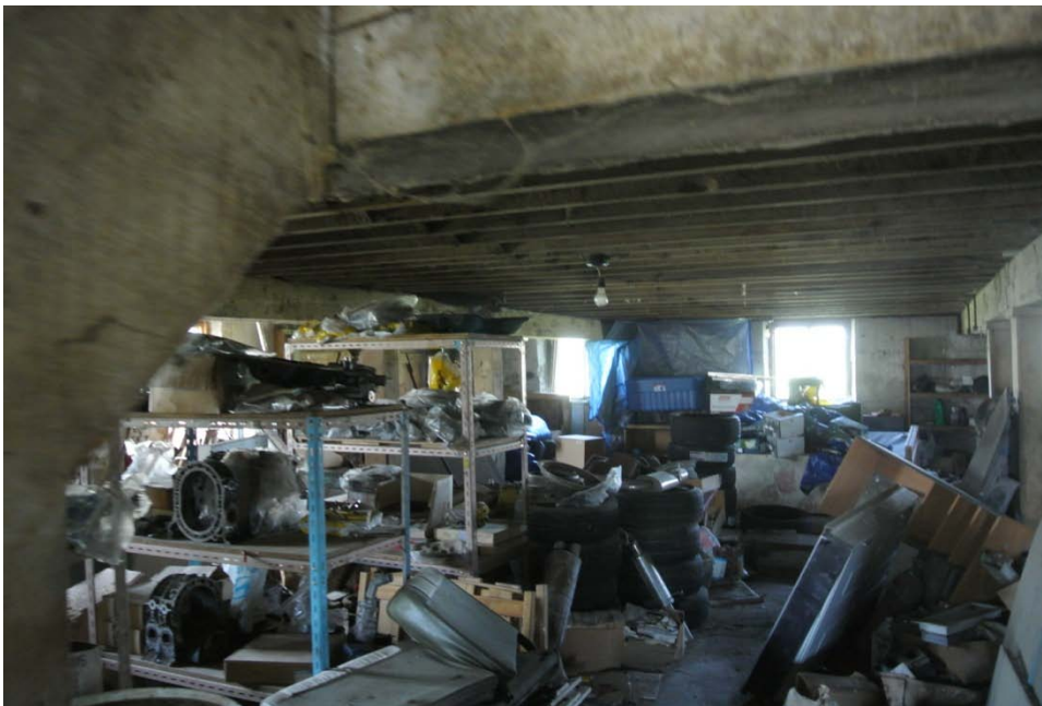
Plate 56: View of the lower level of the barn.
