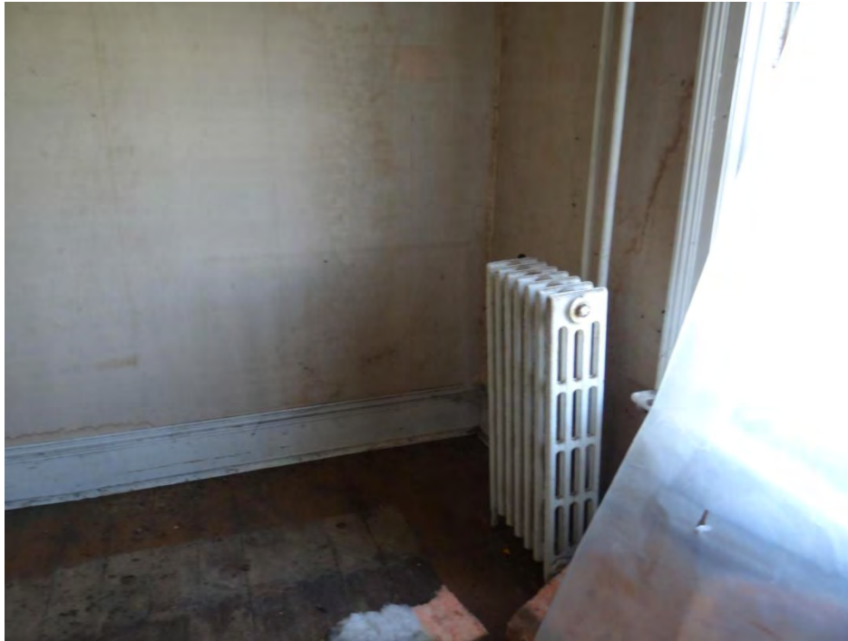
Plate 49: View of the small office on the main floor. Note the moulded baseboards, painted floor boards, cast iron radiator, and moulded window frame.
