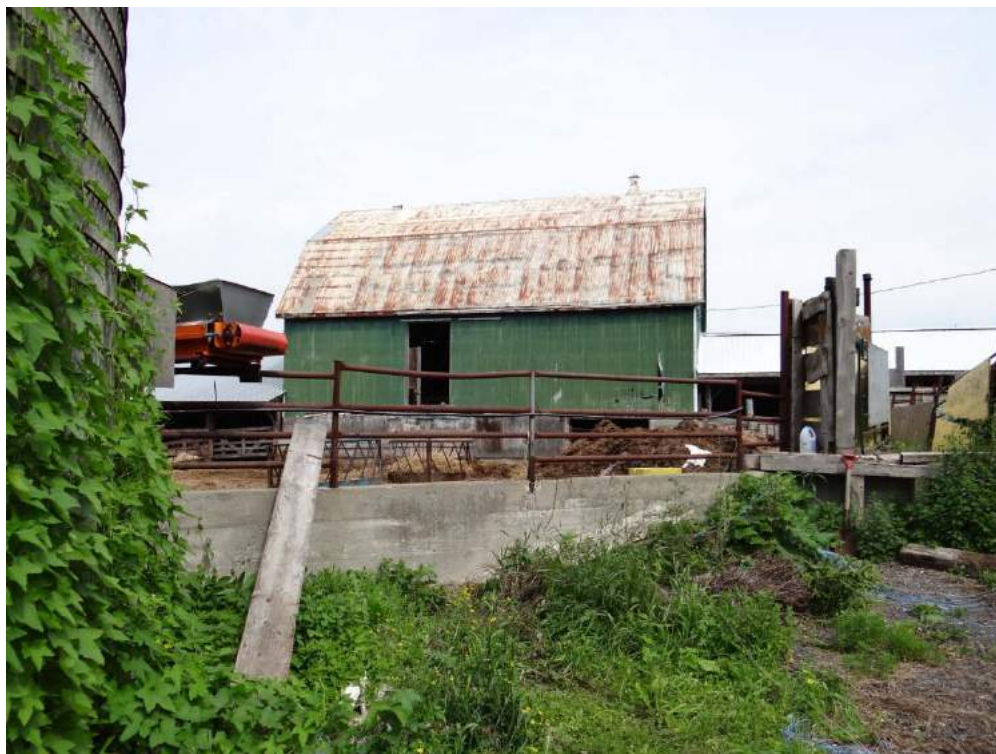
Plate 58: View towards barn.
