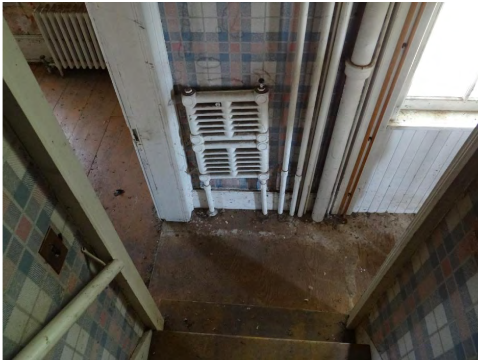
Plate 56: the narrow staircase between living rooms one and two (looking down).
