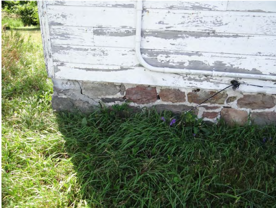
Plate 5: Detail of the stone foundation (northeast corner).
