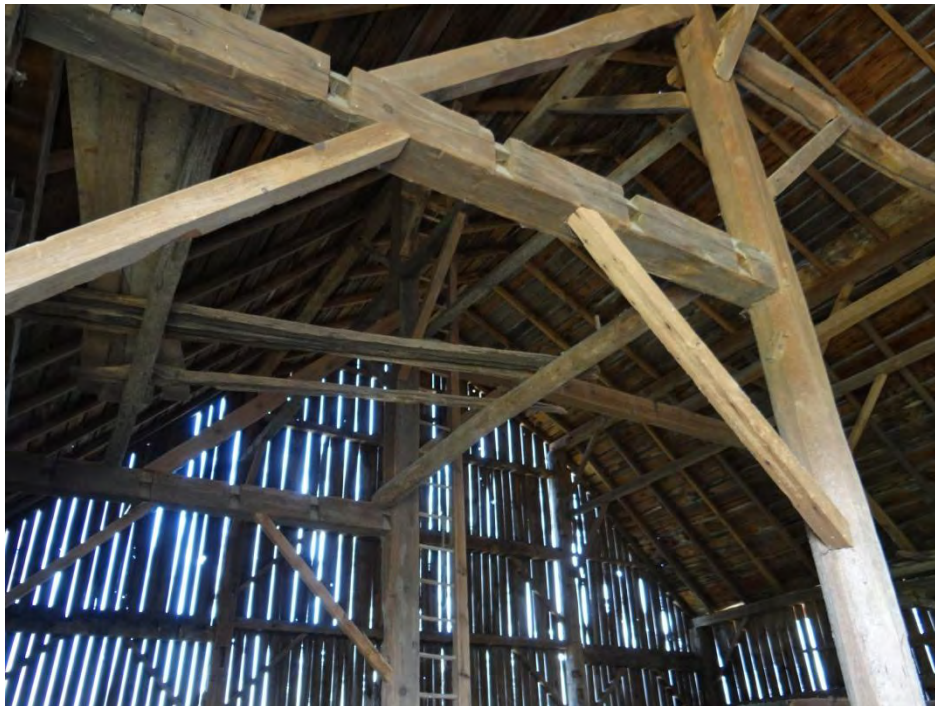
Plate 98: The interior of the barn. Note the hand hewn beams.
