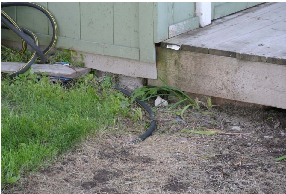
Plate 6: Detail of stone foundations under the northwest corner of the house.
