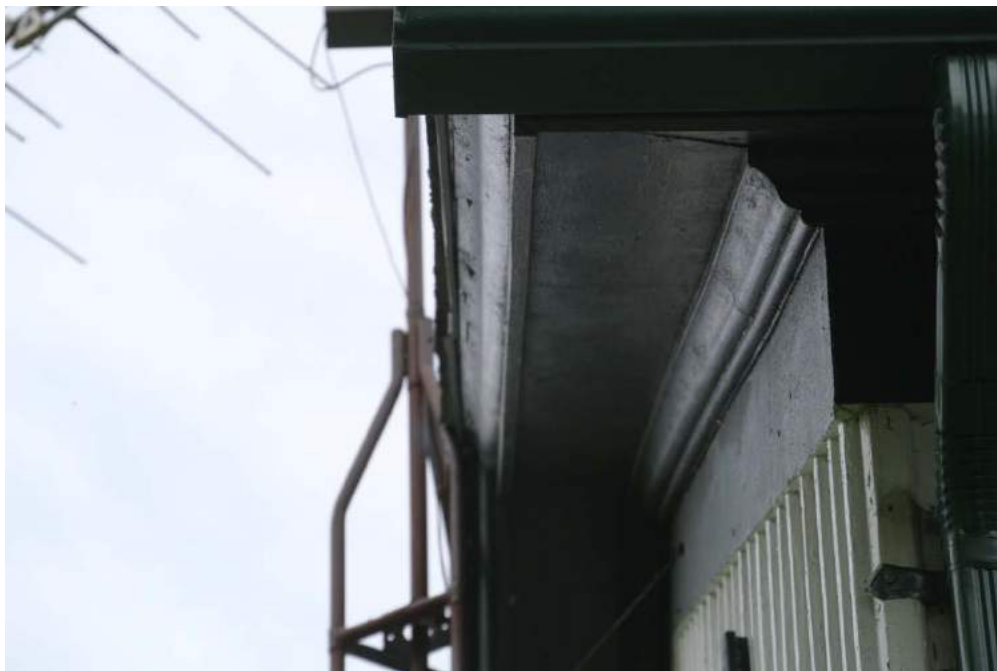
Plate 16: Detail of the wood soffit.
