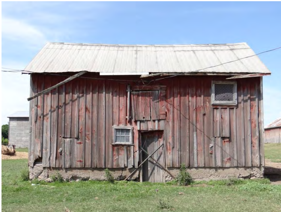
Plate 106: East elevation of the piggery (P). Note the board-and-batten siding and coarse concrete foundations.
