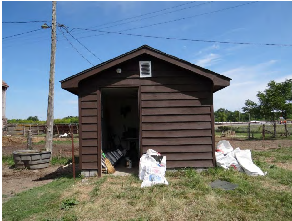
Plate 110: South elevation of outbuilding one (O1).
