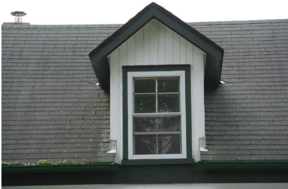
Plate 22: Detail of the dormer on the tail of the original structure.
