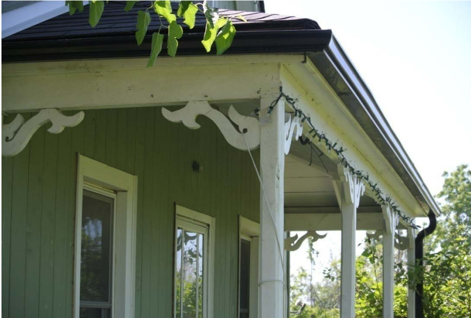
Plate 11: Detail of front verandah, looking south.
