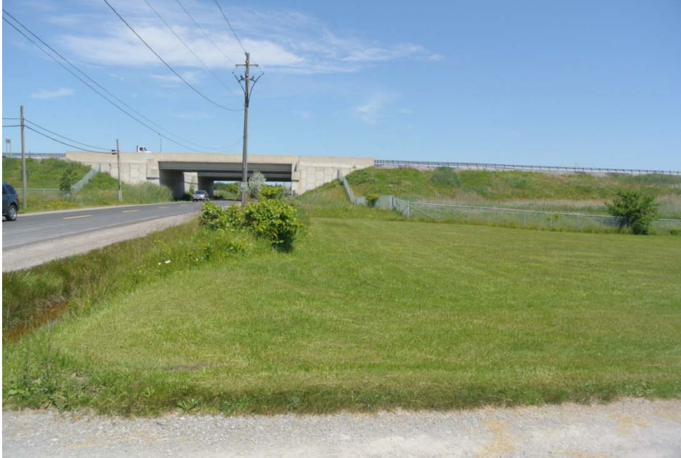
Plate 65: View of the Highway 407 bridge over Reesor Road.
