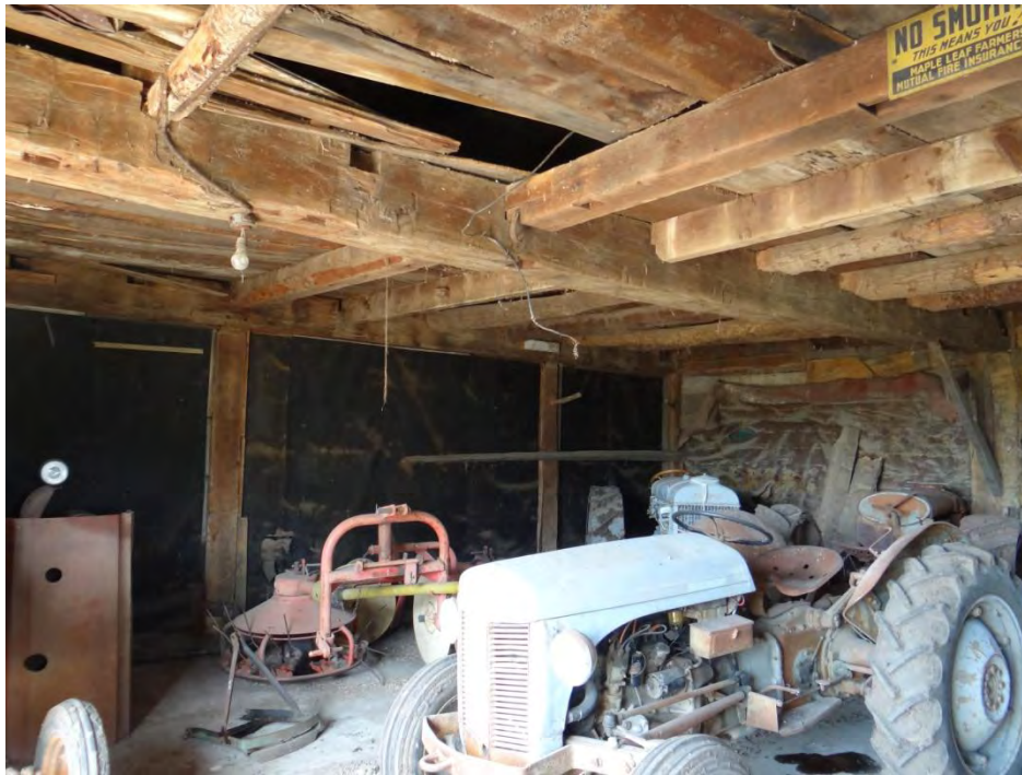
Plate 101: Interior of drive shed one (D1). Note the hand hewn beams.
