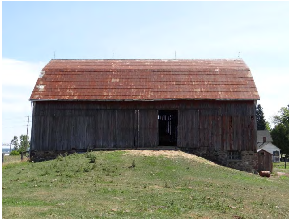
Plate 94: West elevation of the barn.
