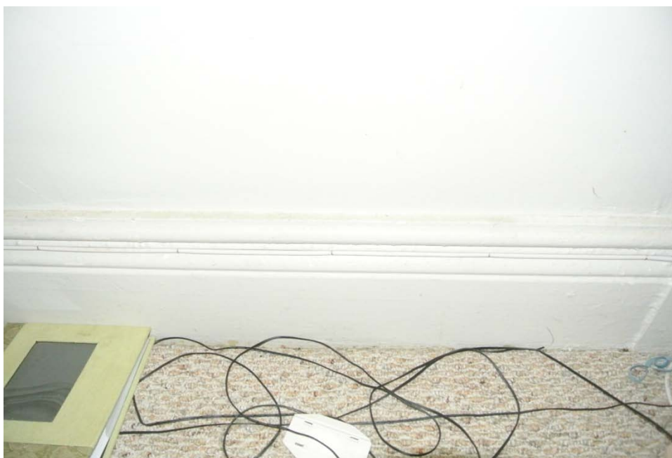
Plate 18: Detail of baseboards in the living room.
