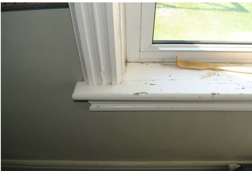
Plate 20: Detail of window casing in main floor bedroom.
