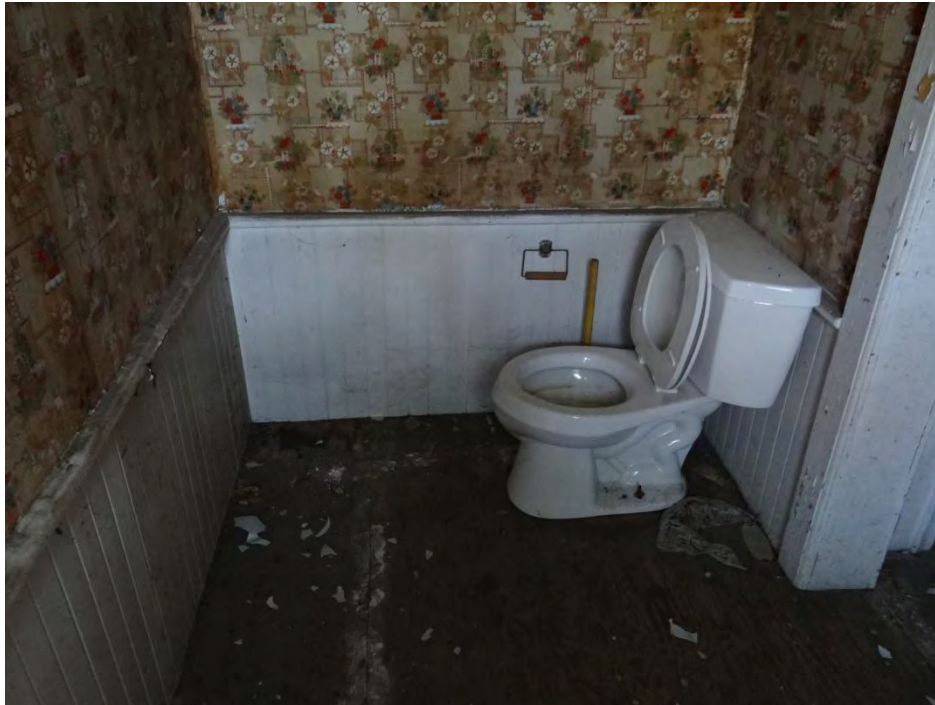
Plate 51: View of the main floor washroom showing the toilet and wainscoting.
