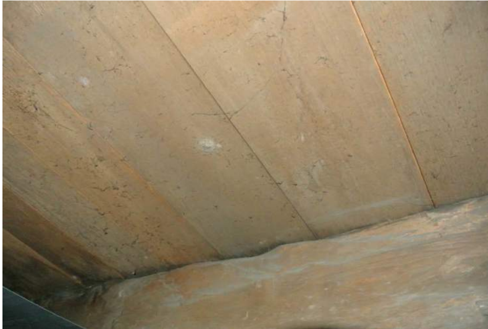
Plate 33: Detail of the first floor floorboards, as seen from the basement.
