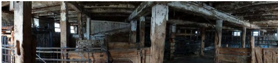
Plate 95: Interior of the barn (lower level).
