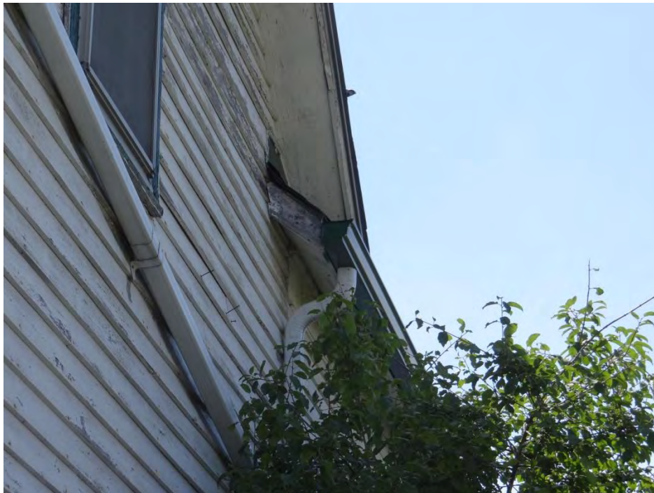
Plate 8: Photo of clapboard siding on the west elevation.
