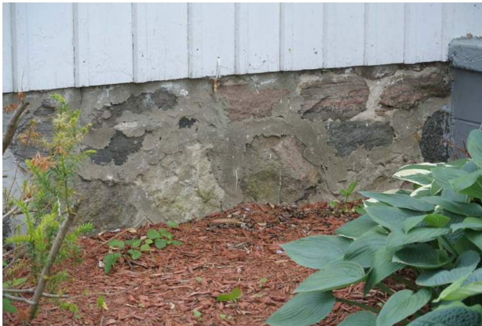
Plate 10: Detail of fieldstone foundations.
