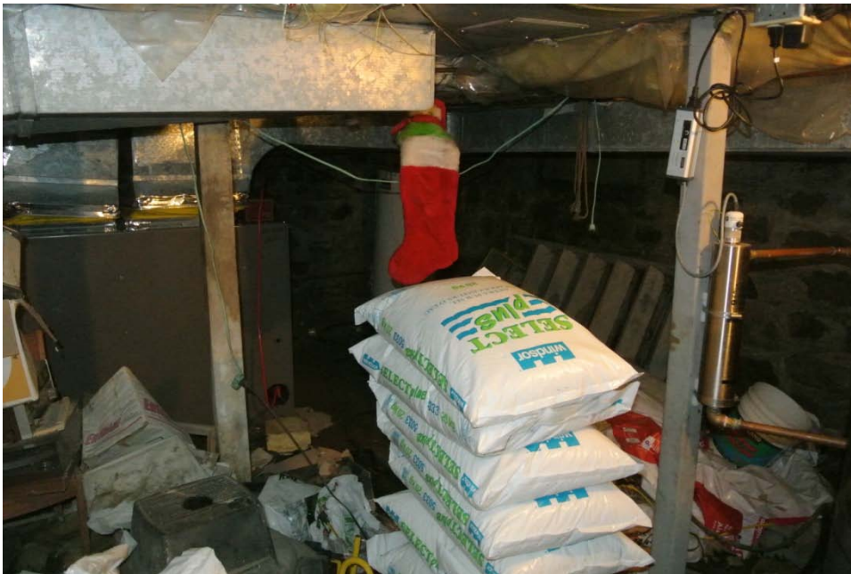
Plate 42: View of the basement from the bottom of the stairs, looking southeast.
