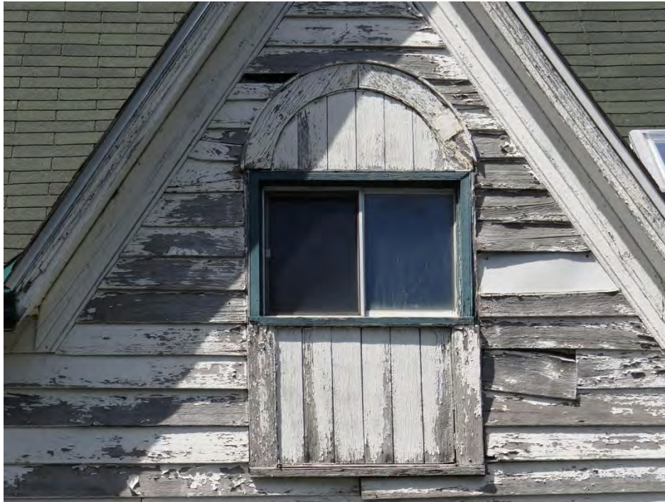
Plate 27: Semi-circular window opening that has been filled and replaced with a modern window.
