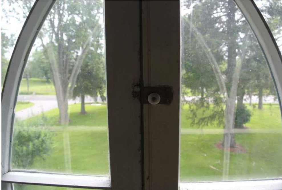
Plate 39: Detail of the arched centrally located, arched window.
