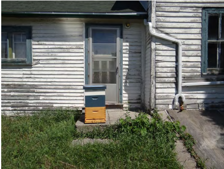
Plate 9: Photo showing the clapboard siding on the south elevation.
