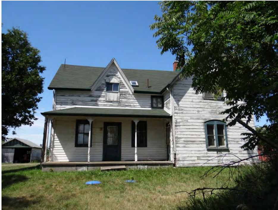
Plate 1: Front facade (east elevation) of the farmhouse.
