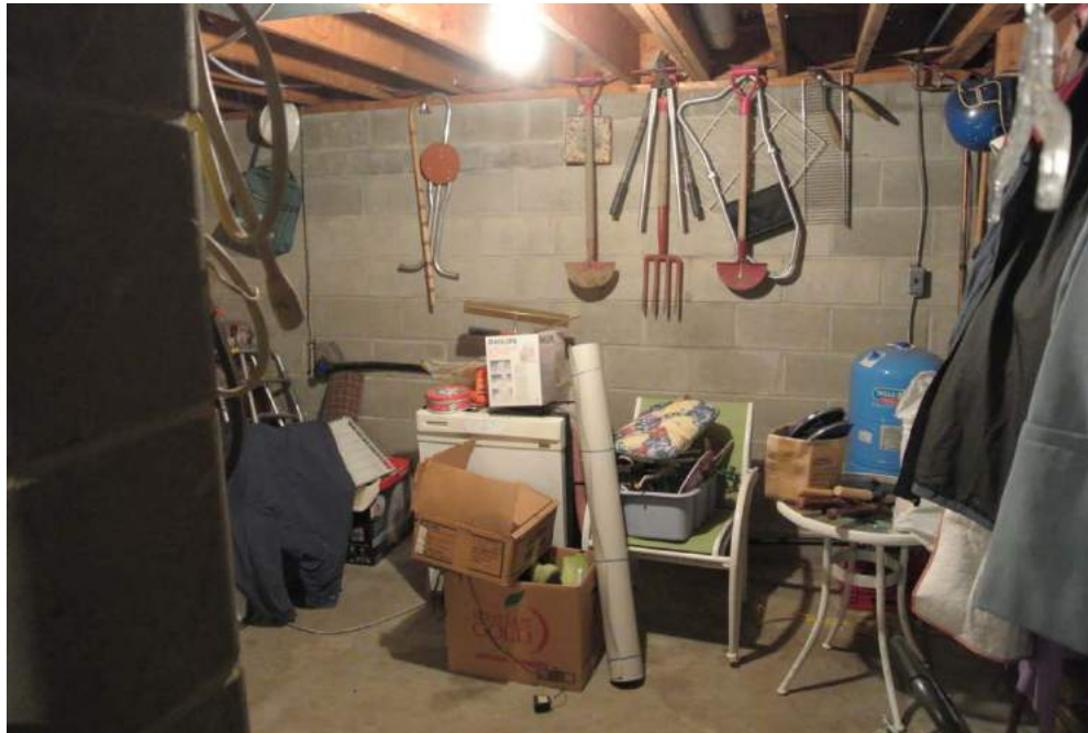
Plate 57: View of basement of modern addition. Note the concrete block foundation, modern cut beams and joists, and poured concrete floor.
