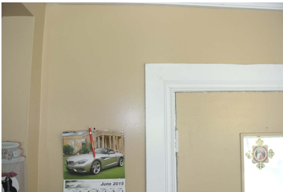
Plate 28: Detail of door casing around side entrance to the kitchen, north wall.
