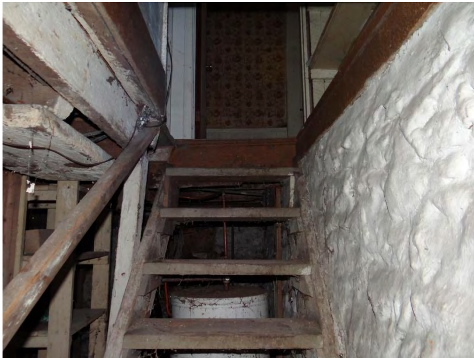
Plate 83: Looking up the basement stairs to the main floor washroom.
