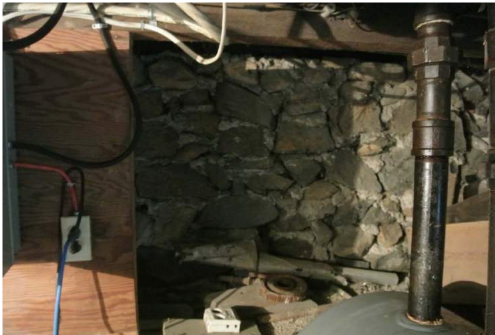
Plate 52. View towards stone foundations located in the basement.
