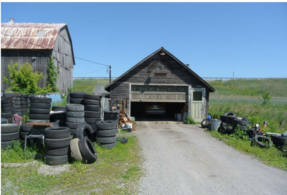
Plate 62: South elevation of the workshop.
