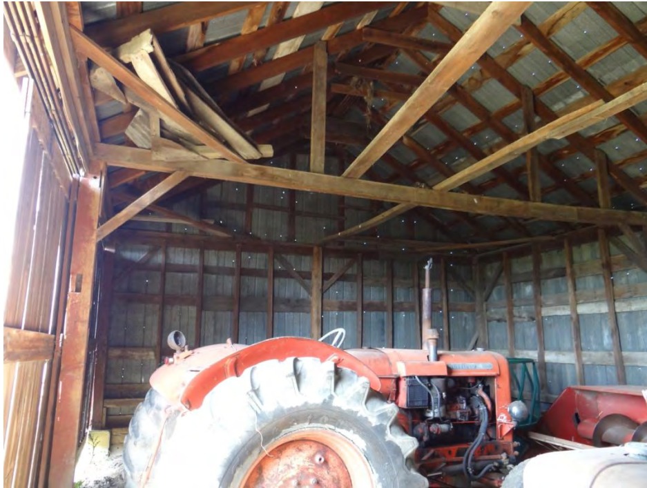
Plate 105: Interior of drive shed three (D3).
