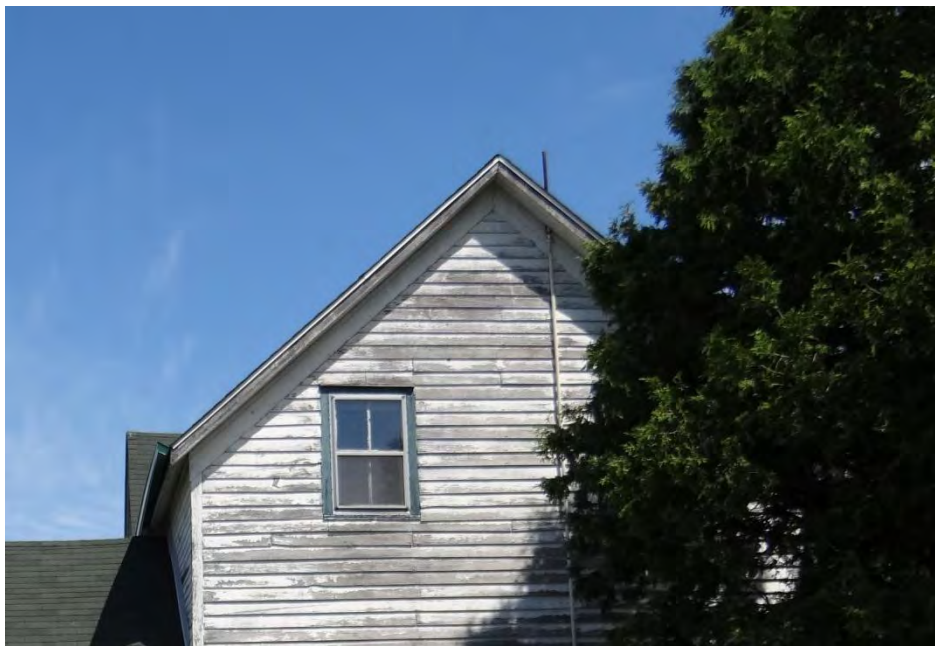
Plate 12: Gable roof on the south section of the residence (south elevation).
