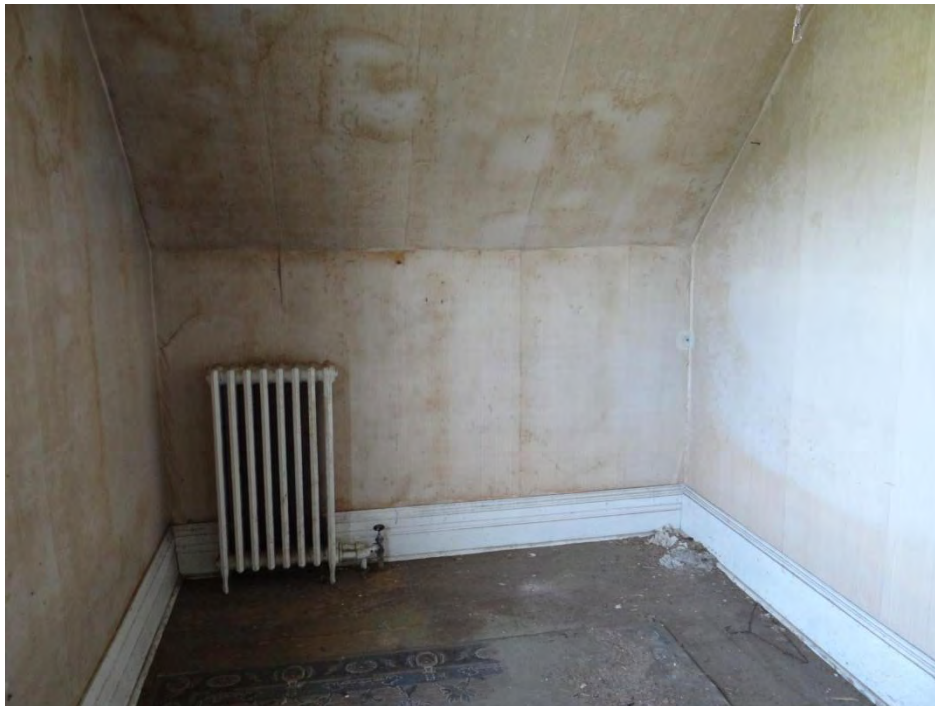
Plate 73: Photo of bedroom three. Note the moulded baseboards and cast-iron radiator.
