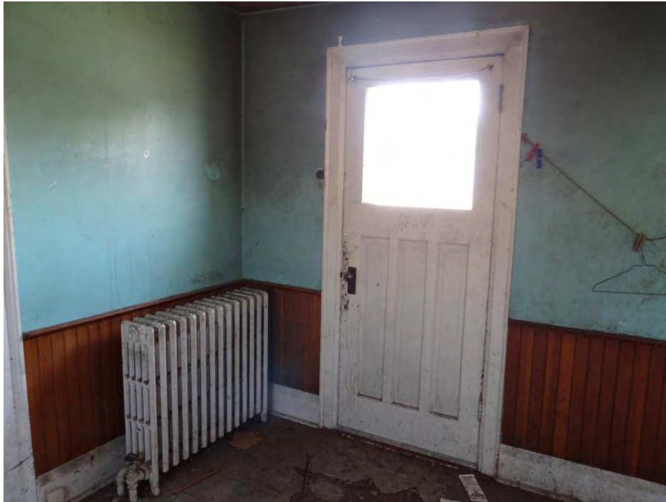
Plate 78: Photo of the exterior door on the south side of the kitchen tail. Note the cast-iron radiator, wainscoting, linoleum floor, and baseboards.
