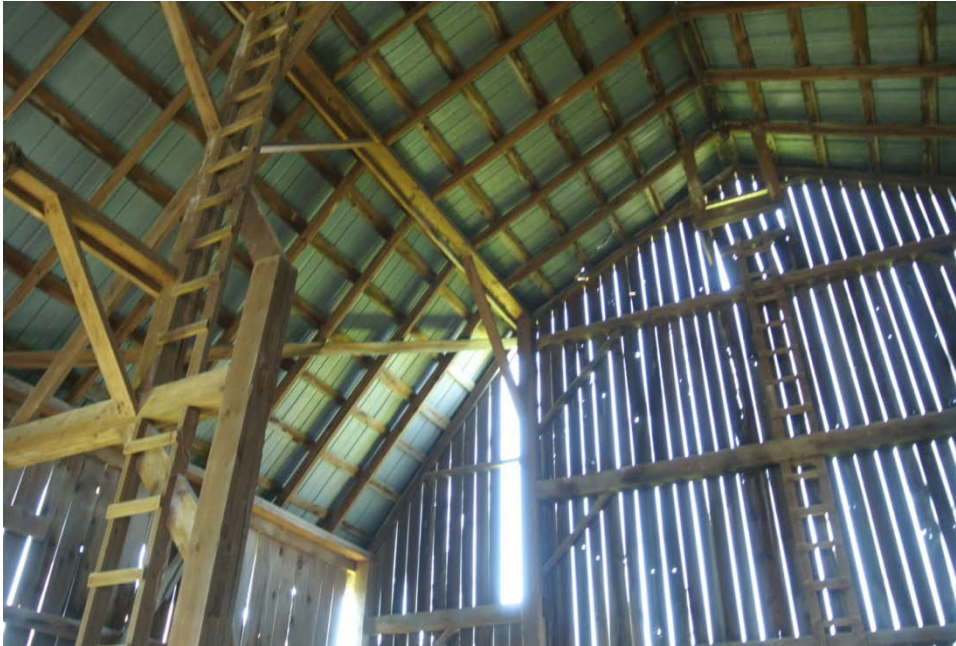
Plate 59: Detail of gambrel roof framing.
