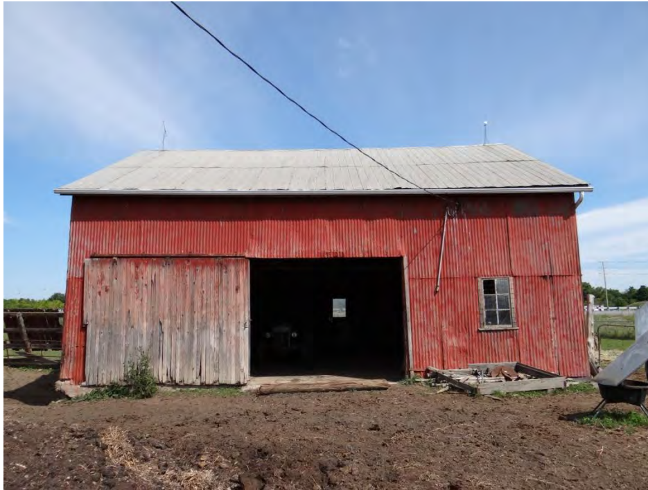
Plate 99: South elevation of drive shed one (D1).
