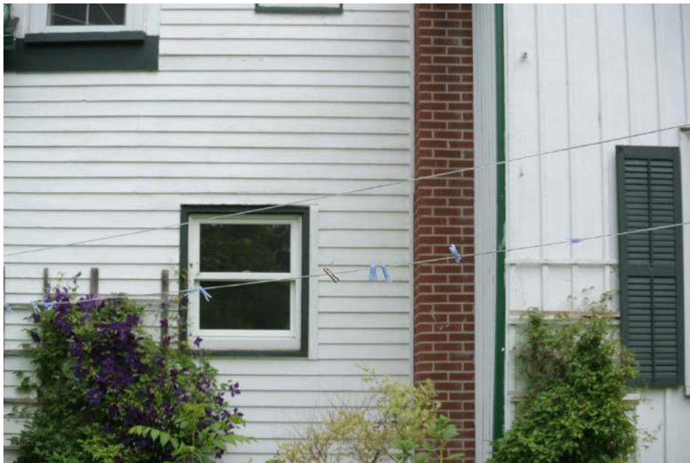
Plate 12: Detail of the chimney located on the south elevation.
