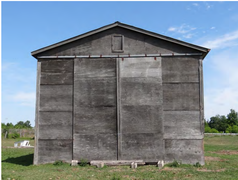
Plate 112: South elevation of outbuilding three (O3).
