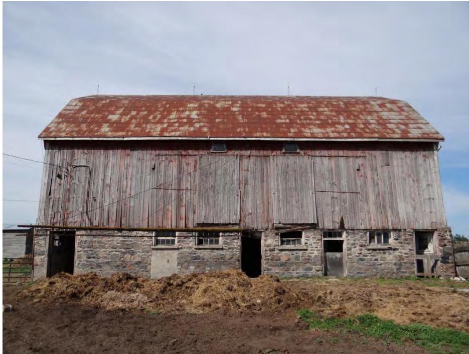
Plate 92: East elevation of the barn.
