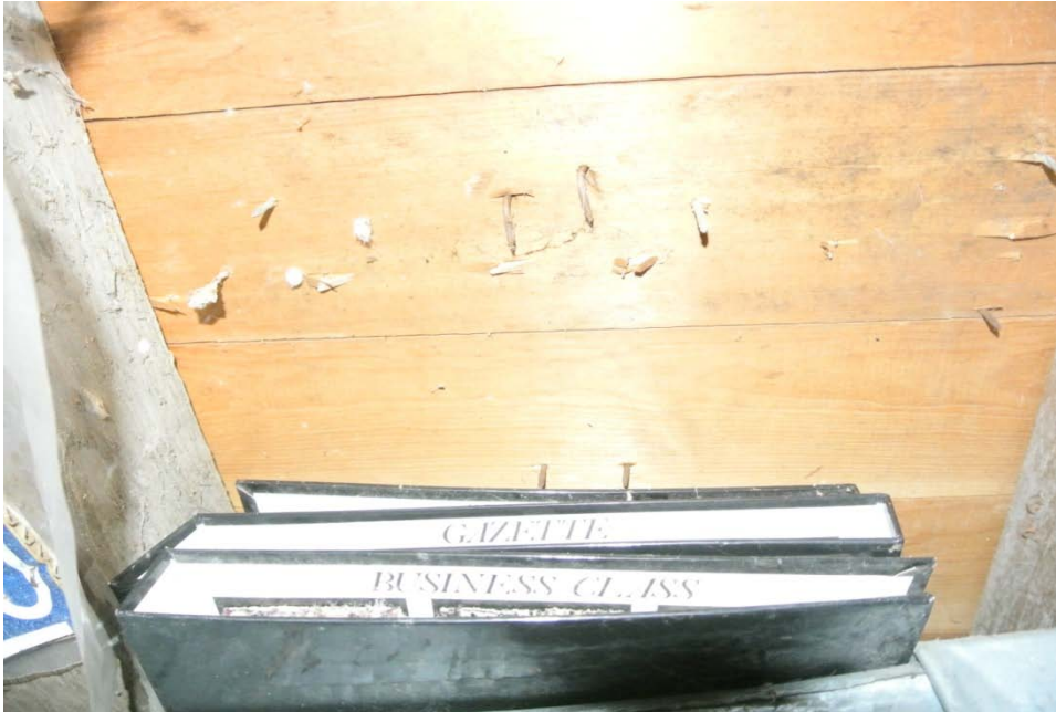
Plate 45: Detail of subfloor above basement.
