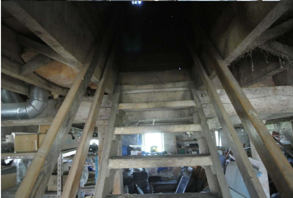
Plate 58: Stairs from the lower level to upper level.
