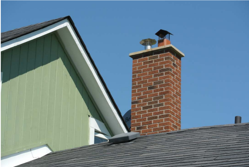
Plate 9: Brick chimney stack located on the north elevation (looking north).
