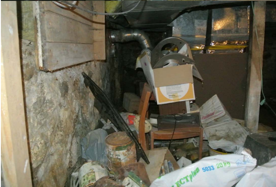
Plate 48: Detail looking east towards northeast corner.
