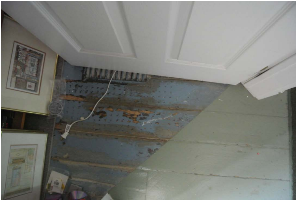
Plate 41: Detail of floor boards and former paint colour, southeast bedroom.
