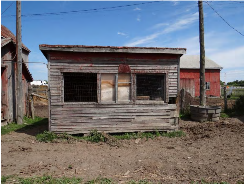
Plate 109: South elevation of the chicken coop (C).
