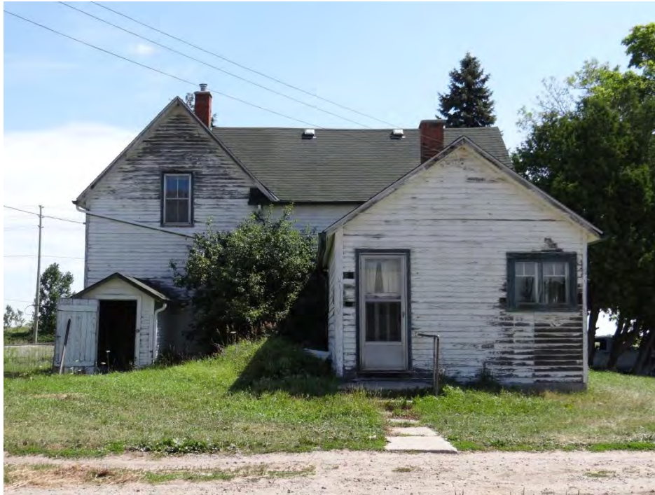
Plate 3: West elevation of the farmhouse.
