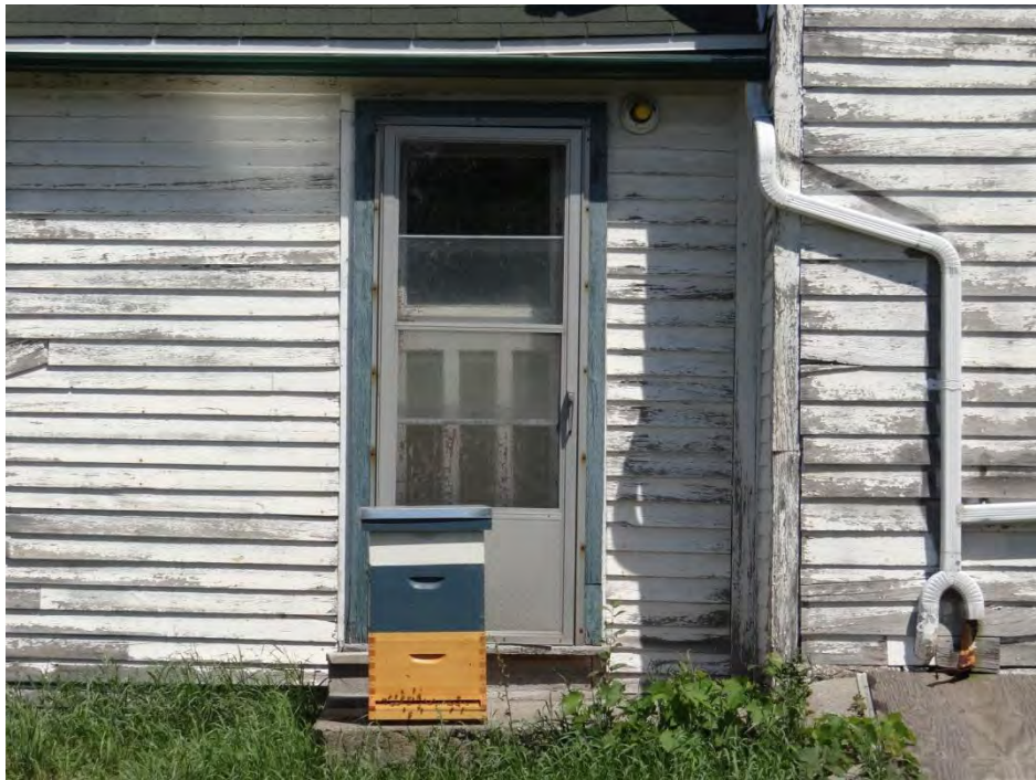
Plate 20: Door on the south elevation.
