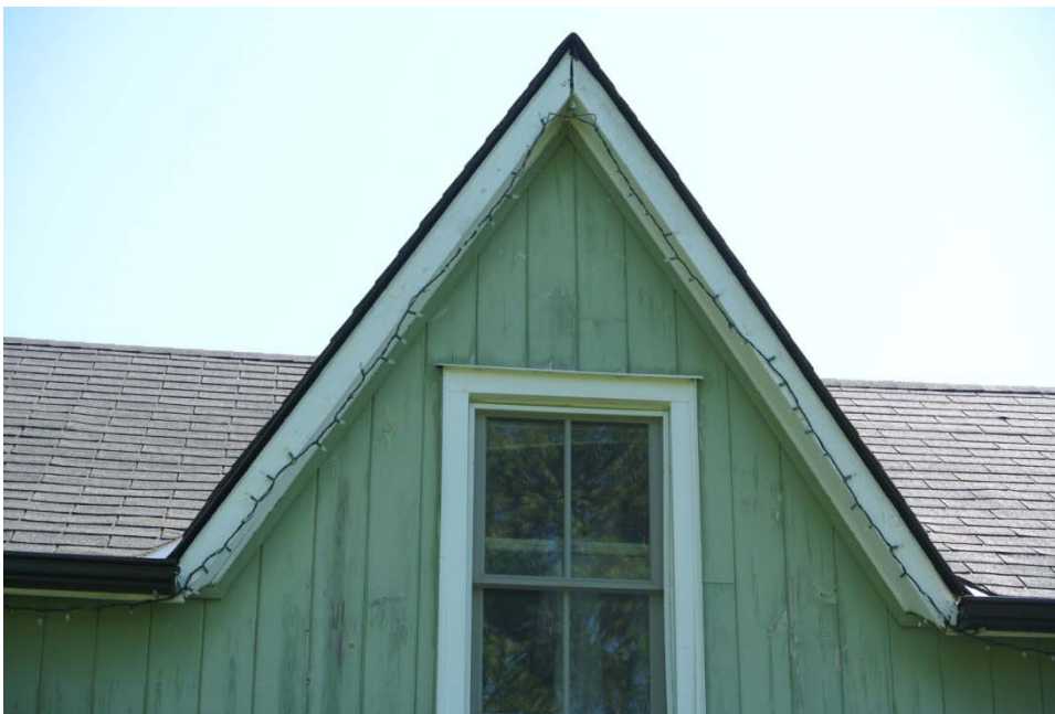
Plate 10: Detail of central gable dormer and two-over-two pane sash window.
