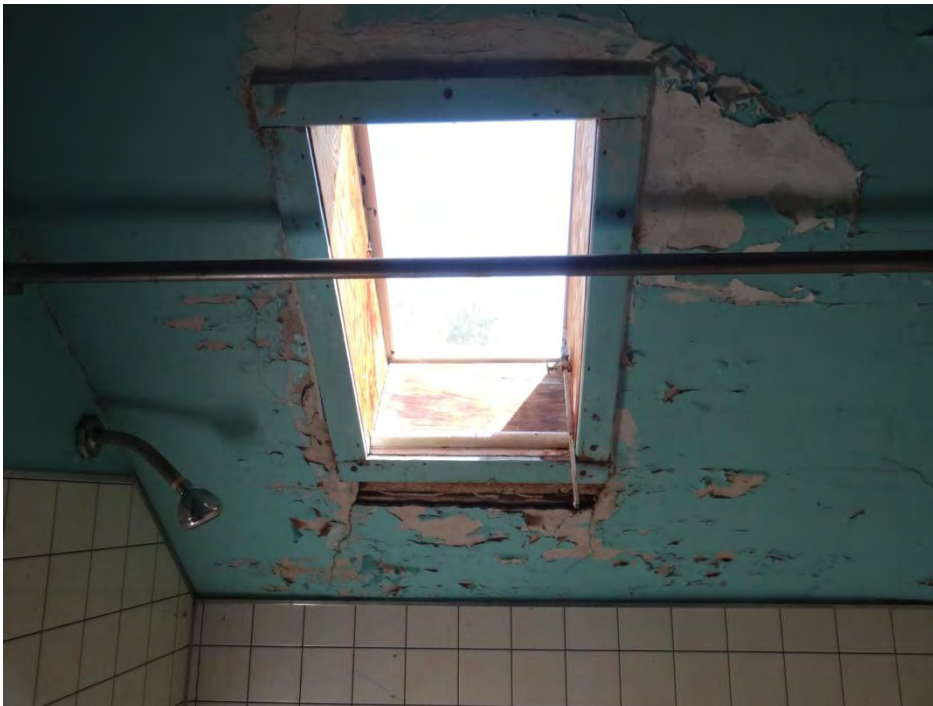
Plate 64: The skylight in the second floor washroom.
