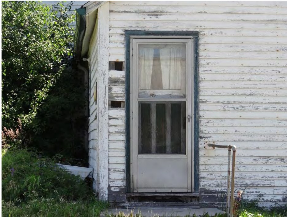
Plate 21: Door leading to the kitchen, west elevation.
