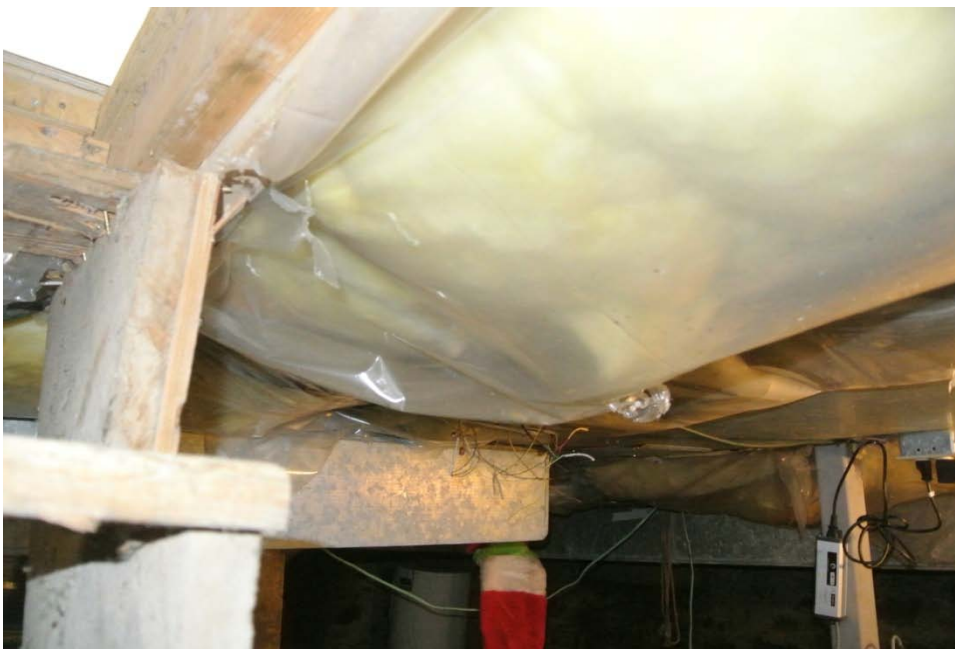
Plate 46: Detail of basement ceiling. Note insulation and ductwork.
