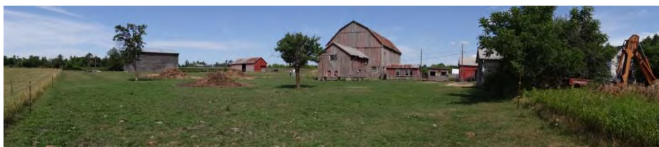
Plate 115: Northeast view of the property showing the outbuildings and barn.
