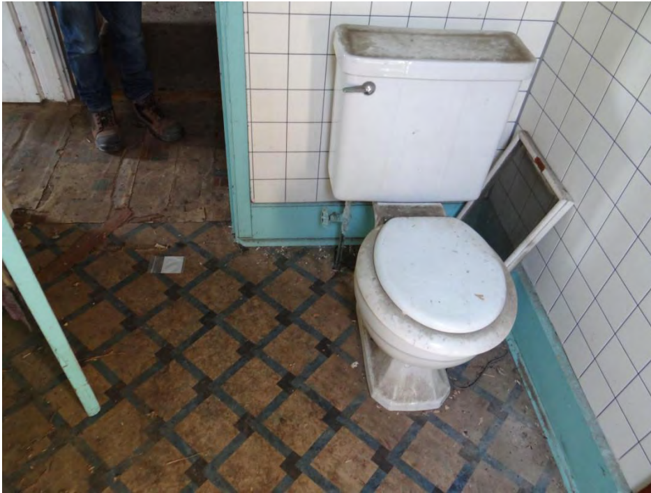
Plate 63: The second floor washroom looking towards the hallway.
