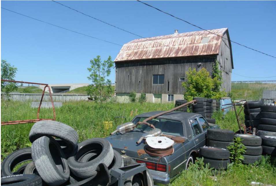
Plate 51: View of the south and east elevations of the barn.
