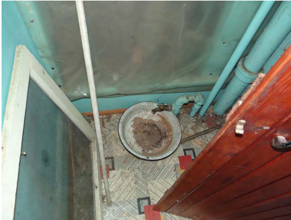
Plate 67: The faucet and water pan second floor washroom closet. Use unknown.
