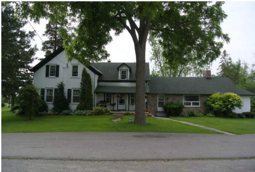
Plate 4: North elevation of residence.
