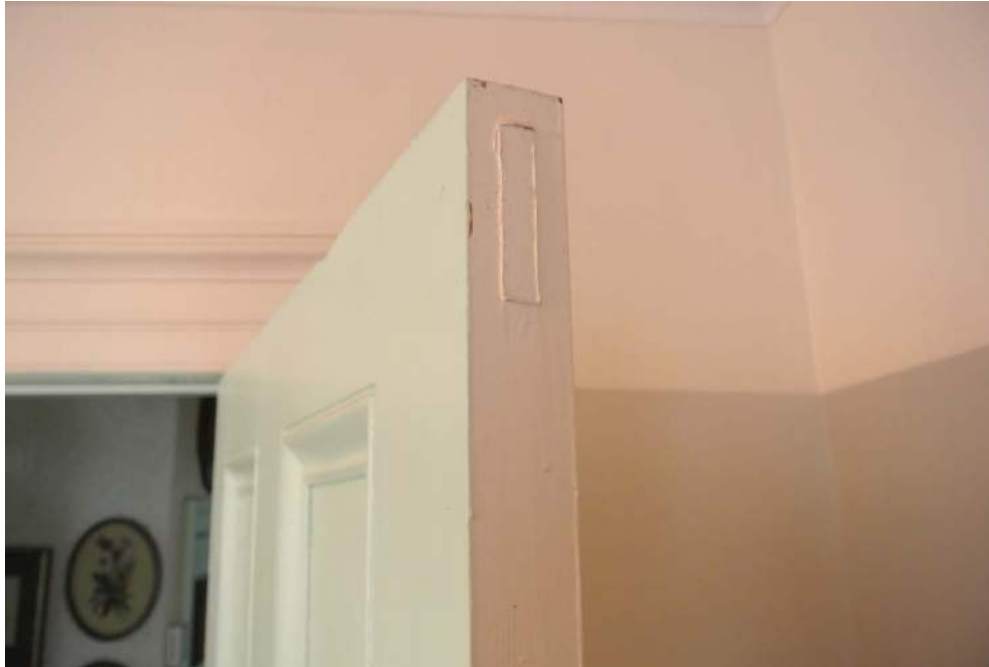
Plate 29: Detail of original door located on the first floor.
