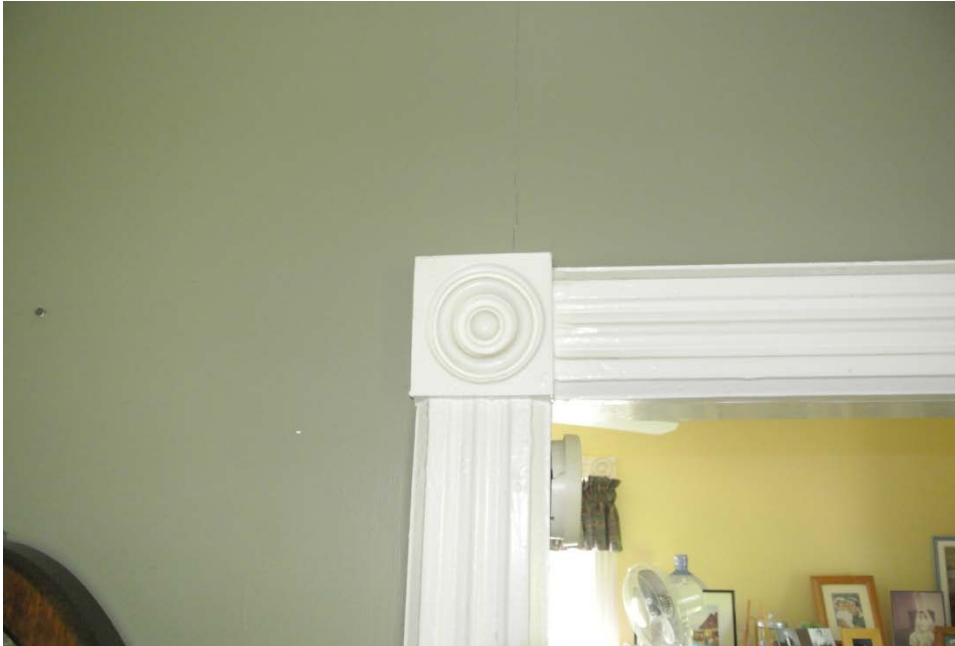
Plate 21: Detail of door casing and corner rosette block, living room.
