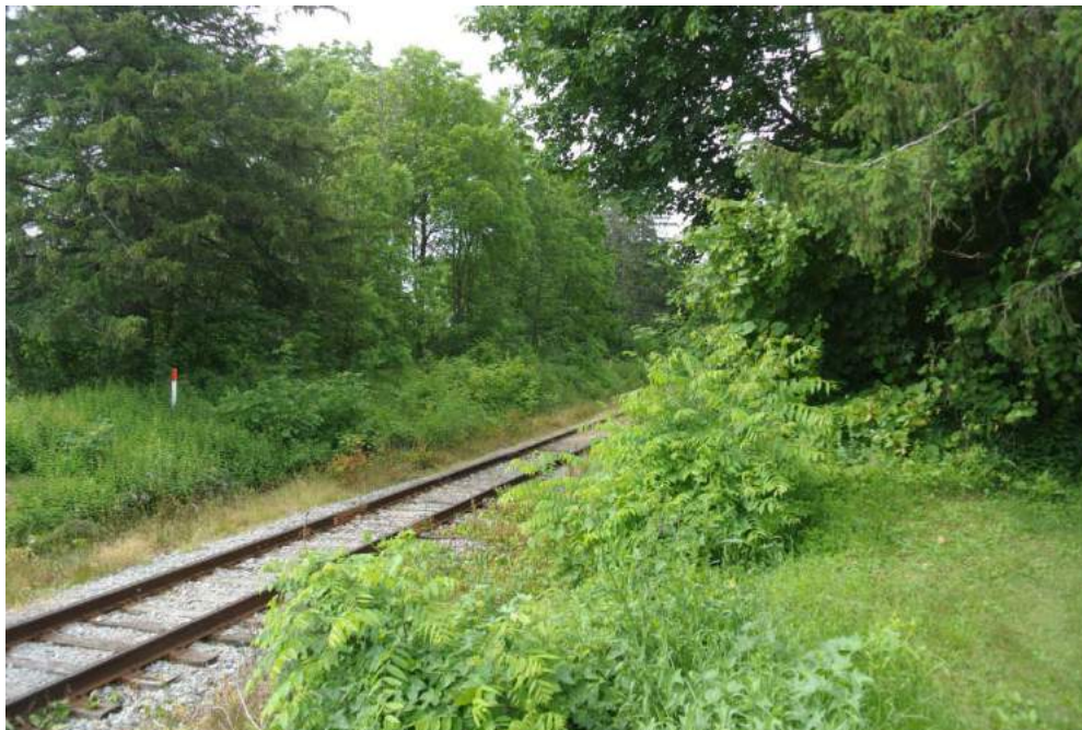
Plate 66: View towards the CPR line to the south of the property.
