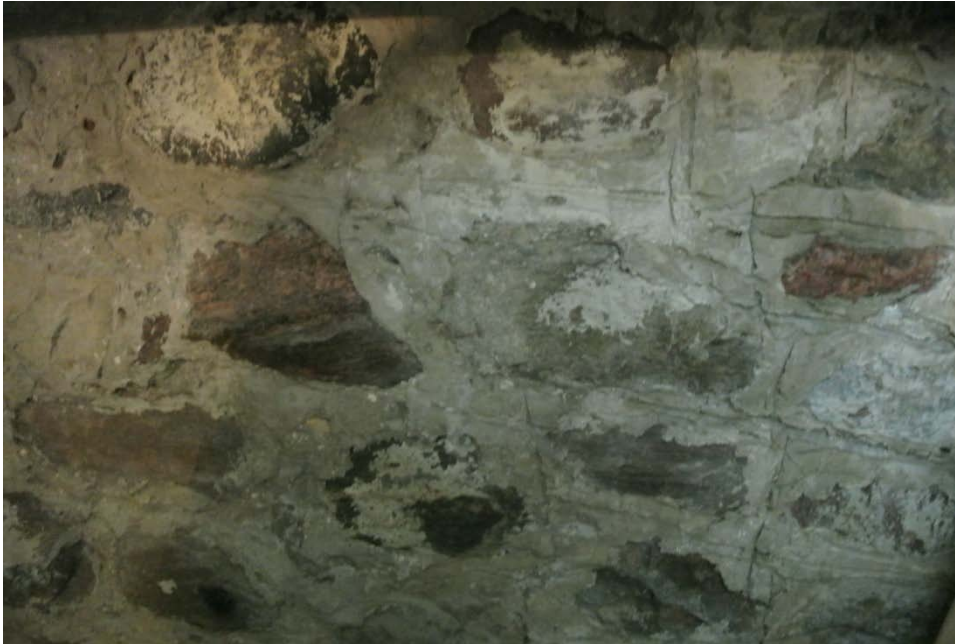
Plate 43: Detail of stone foundation walls.
