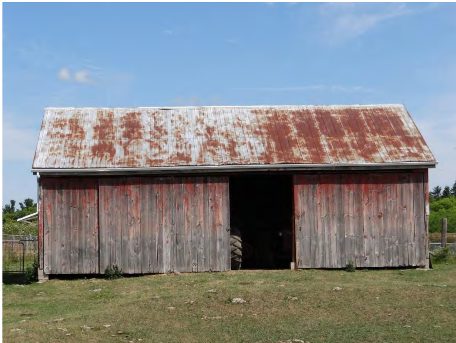
Plate 104: South elevation of drive shed three (D3).
