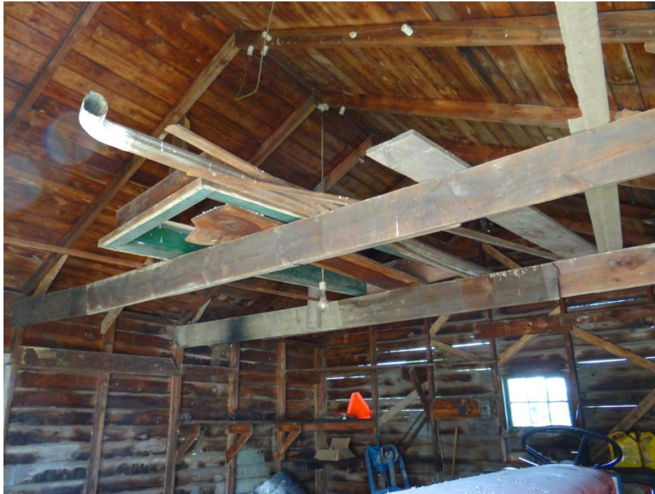
Plate 103: The interior of D2 showing relatively new beams and construction techniques.
