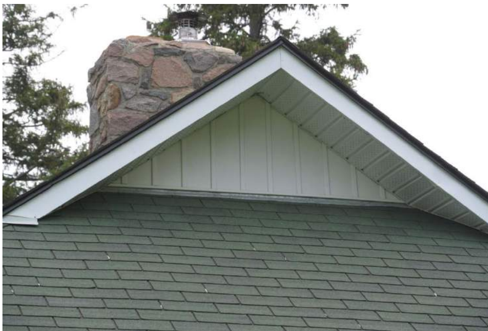
Plate 20: Detail of the 'Dutch Gable' roof and stone chimney.
