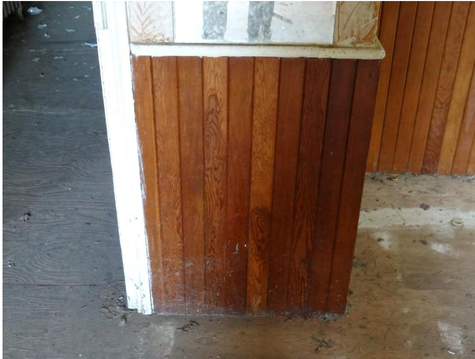
Plate 32: Photo of the wainscoting in living room one.
