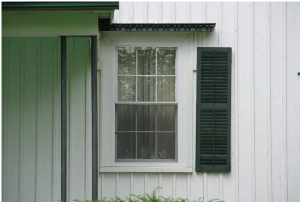
Plate 6: Detail of lintel over window on north elevation.
