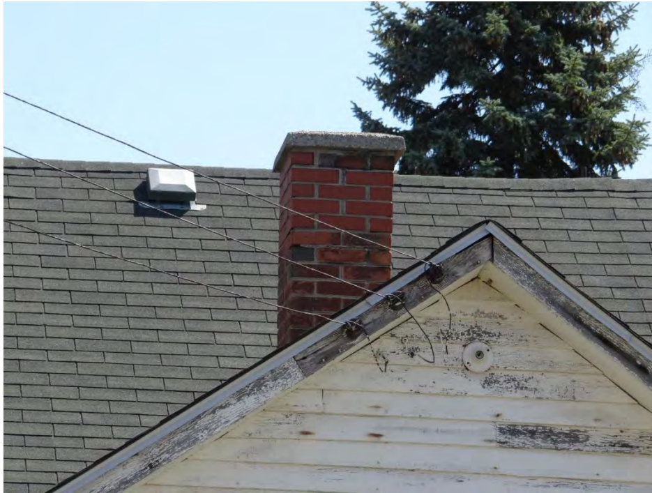
Plate 17: Photo of the interior, red brick chimney located in the kitchen tail.
