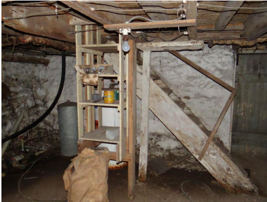
Plate 82: Photo of the basement under the original south section of the house looking towards the stairs that lead to the main floor washroom.
