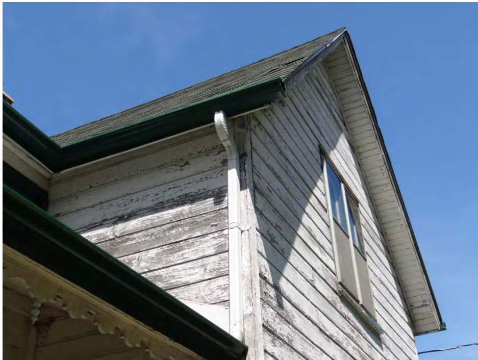
Plate 6: Photo of the shiplap cladding on the east and south elevations.
