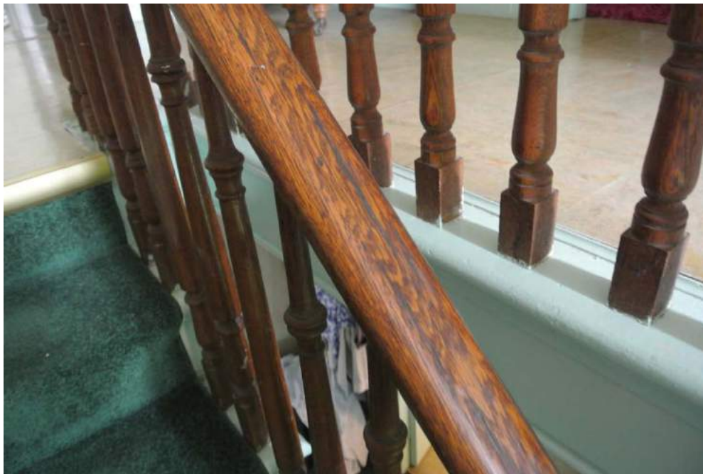
Plate 28: Detail of the staircase railing.
