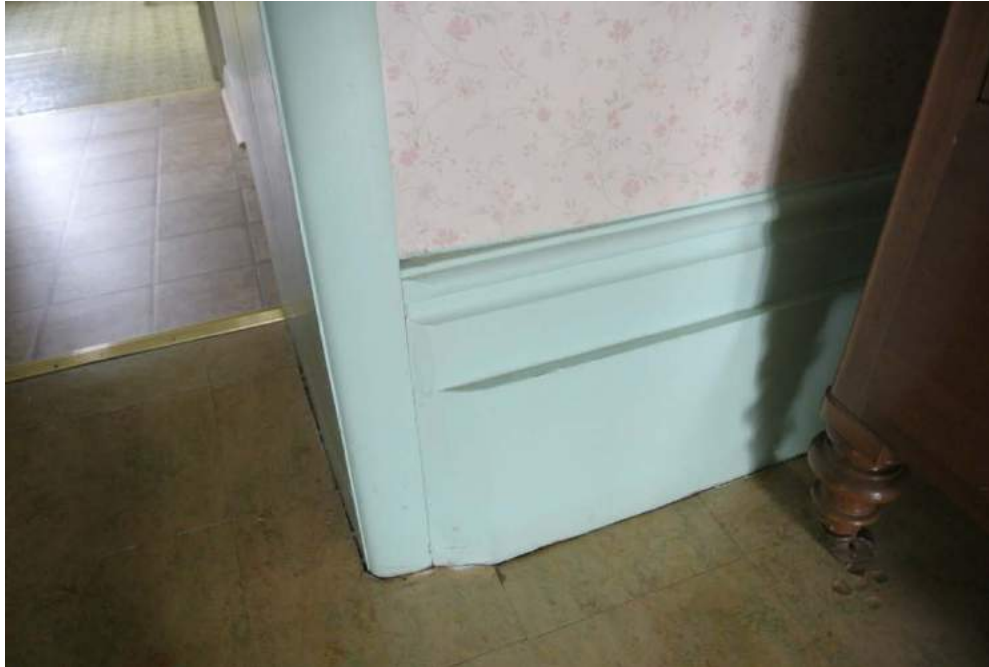
Plate 45: Detail of baseboards located in upstairs hallway.
