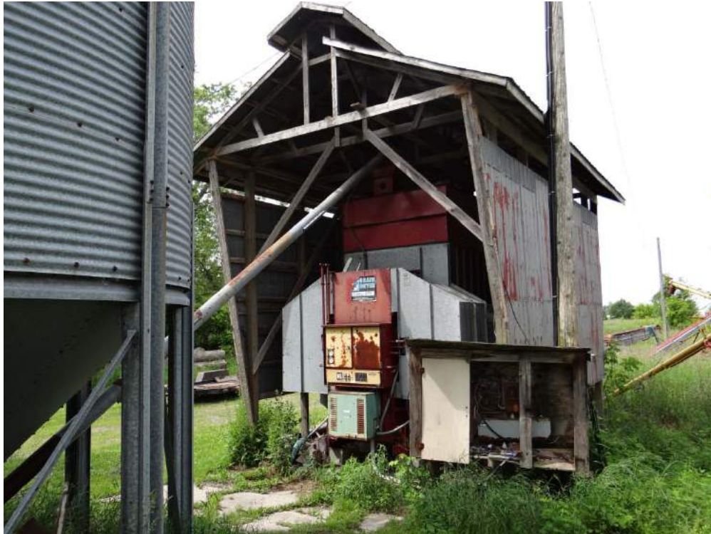
Plate 63: View towards Outbuilding 1, located in the granary complex.
