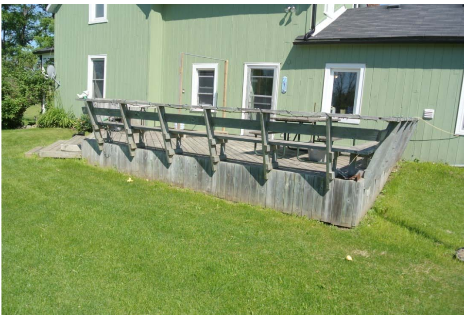
Plate 14: View of modern raised deck on the south elevation.
