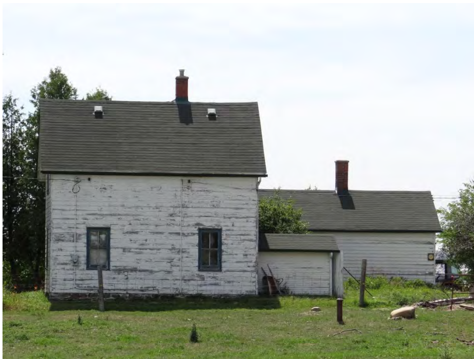
Plate 4: North elevation of the farmhouse.
