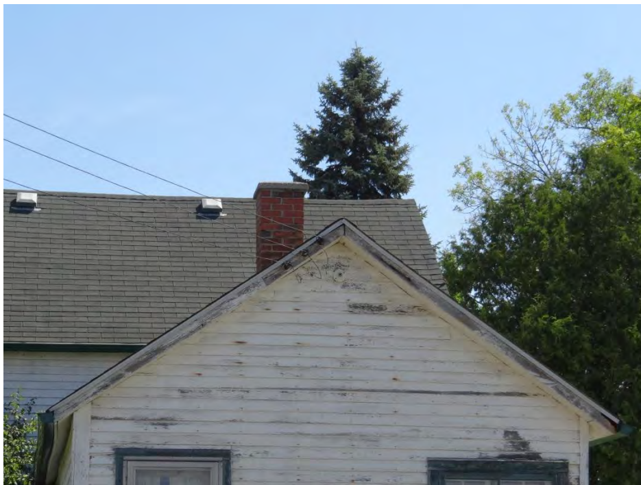
Plate 14: Gable roof of the kitchen tail (west elevation).
