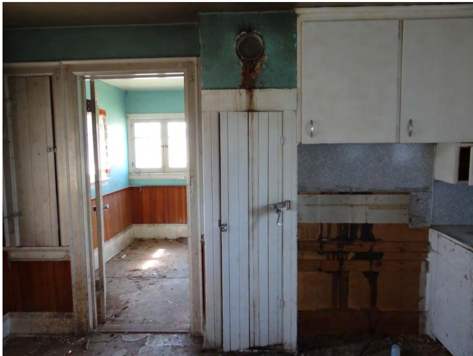
Plate 79: Photo of the kitchen tail looking towards the mud room.
