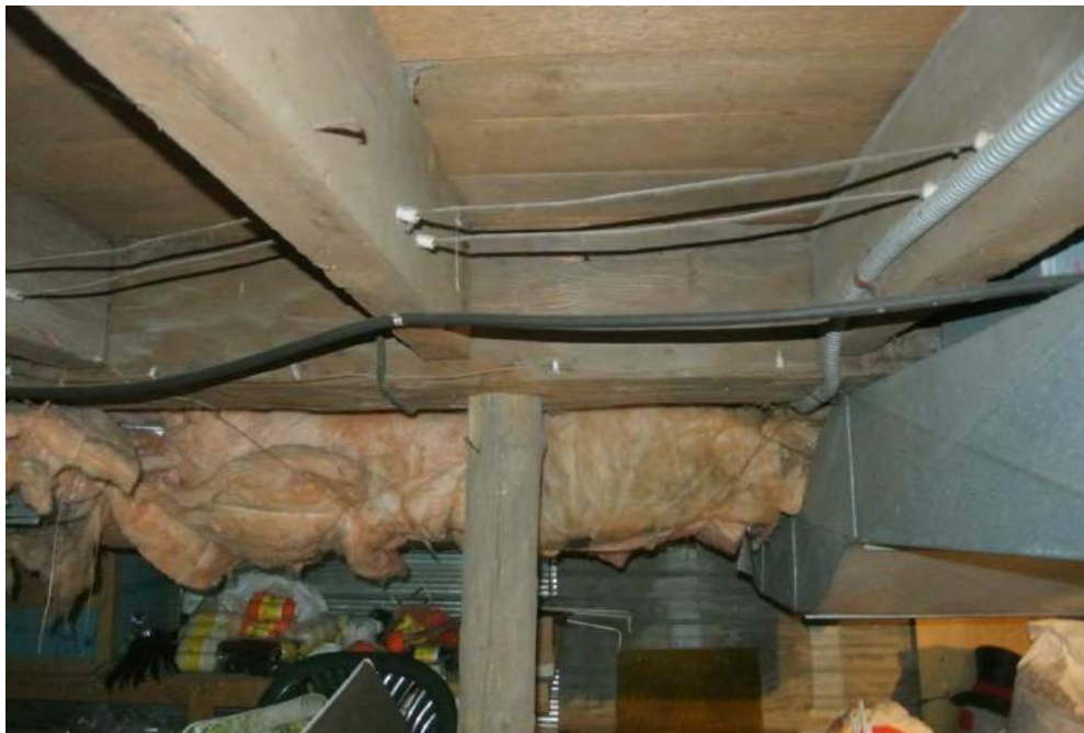
Plate 54: Detail of the hewn beams and milled joists.
