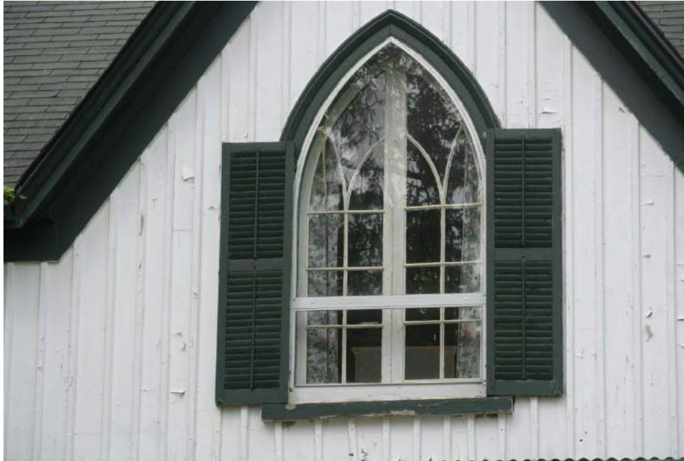
Plate 9: Detail of Gothic arched window.
