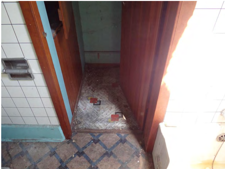
Plate 66: The closet in the second floor washroom.
