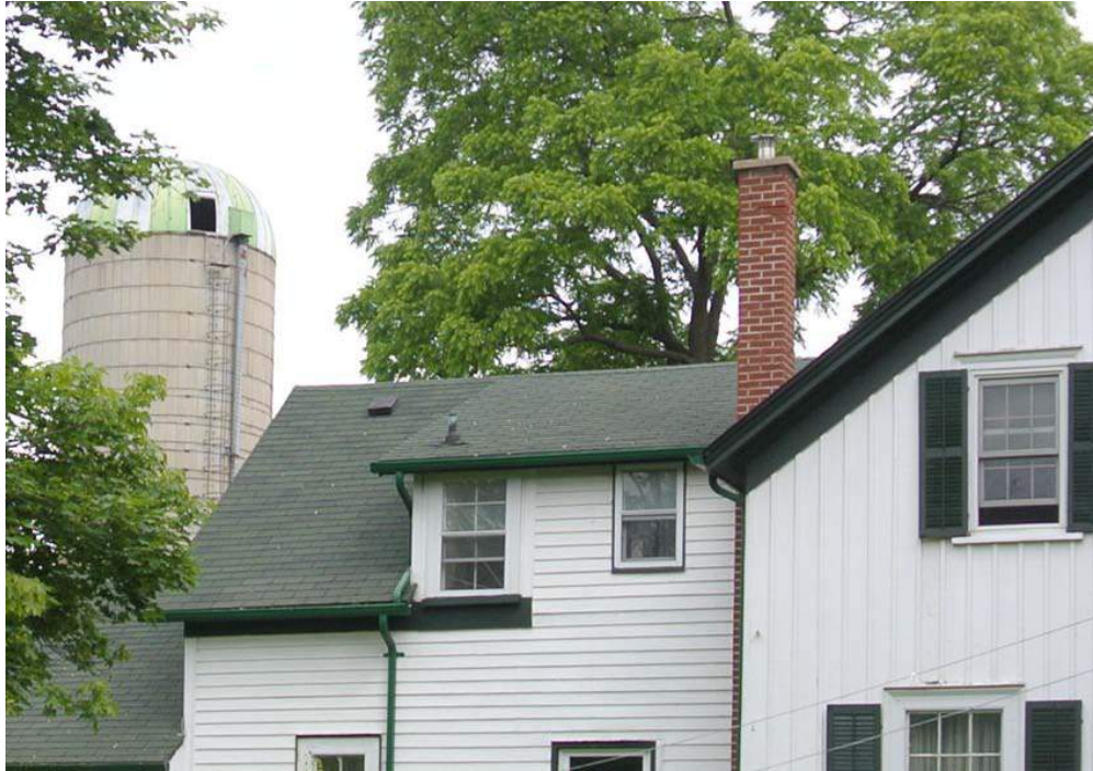
Plate 15: View towards the tail of the original structure.
