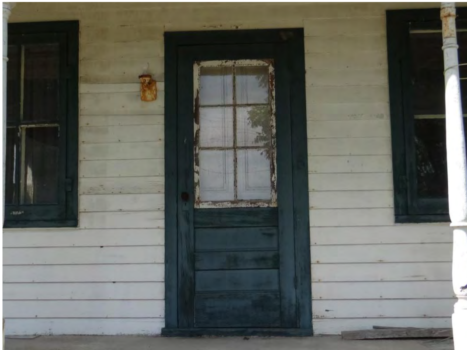
Plate 18: Door on the front façade (east elevation).
