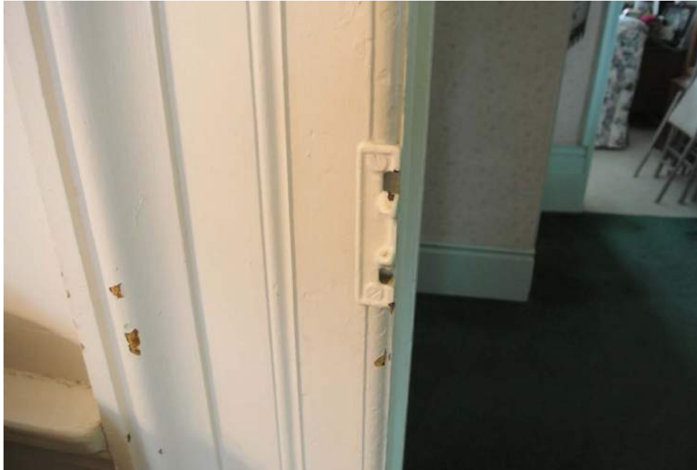
Plate 31. Detail of hardware located on the doorway of a first-floor door.
