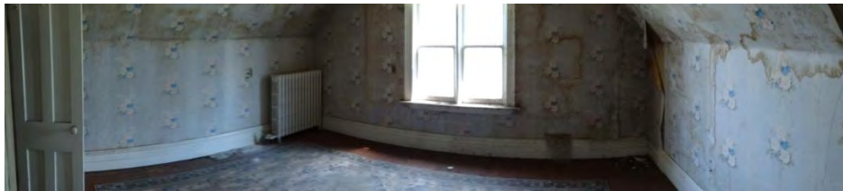
Plate 68: View of bedroom two from the hallway door.
