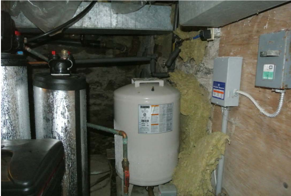
Plate 47: Basement, looking south towards southwest corner.
