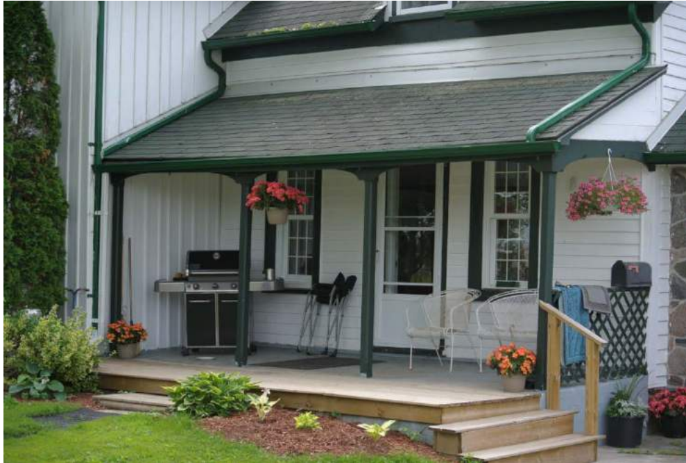
Plate 23: View towards the veranda on the north elevation.
