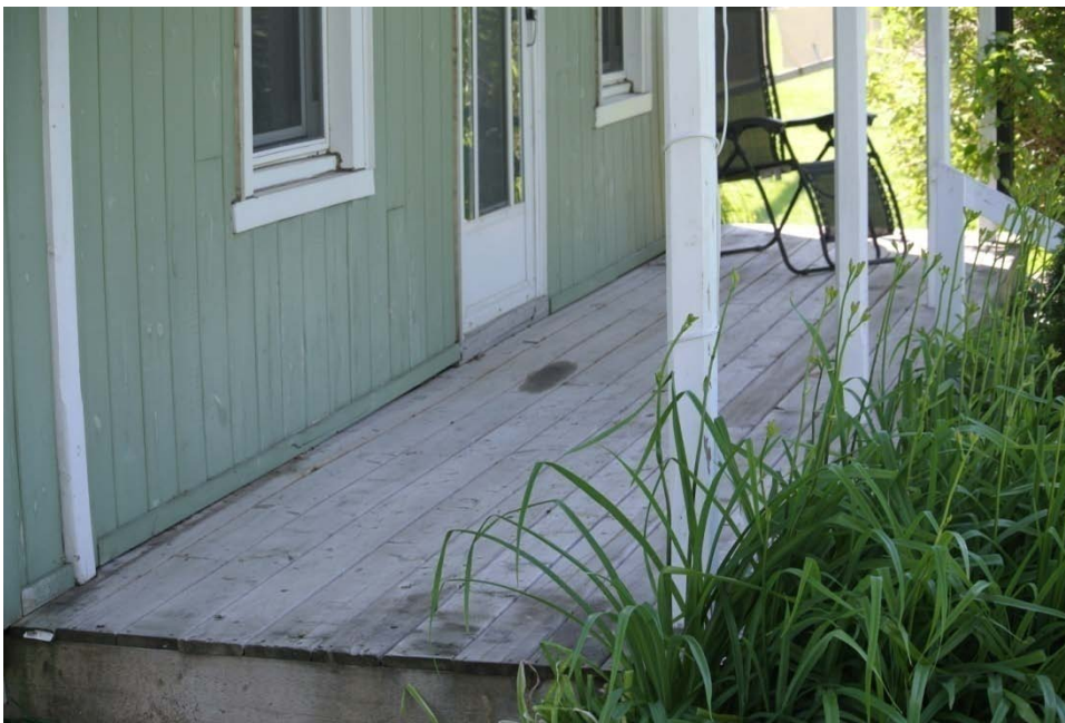
Plate 12: Detail of front verandah, looking south.
