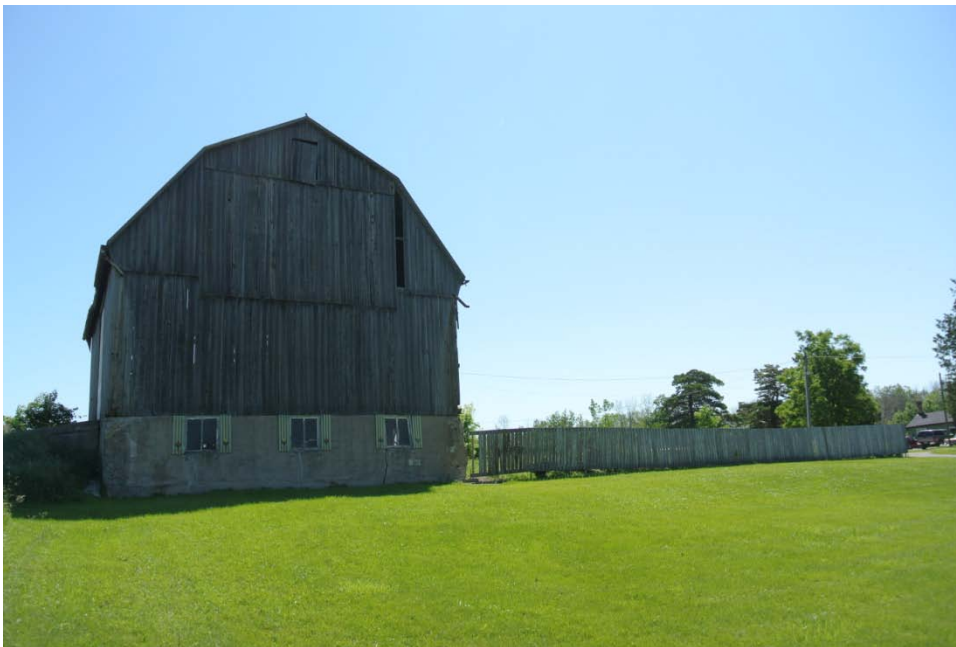
Plate 54: East elevation of the barn.
