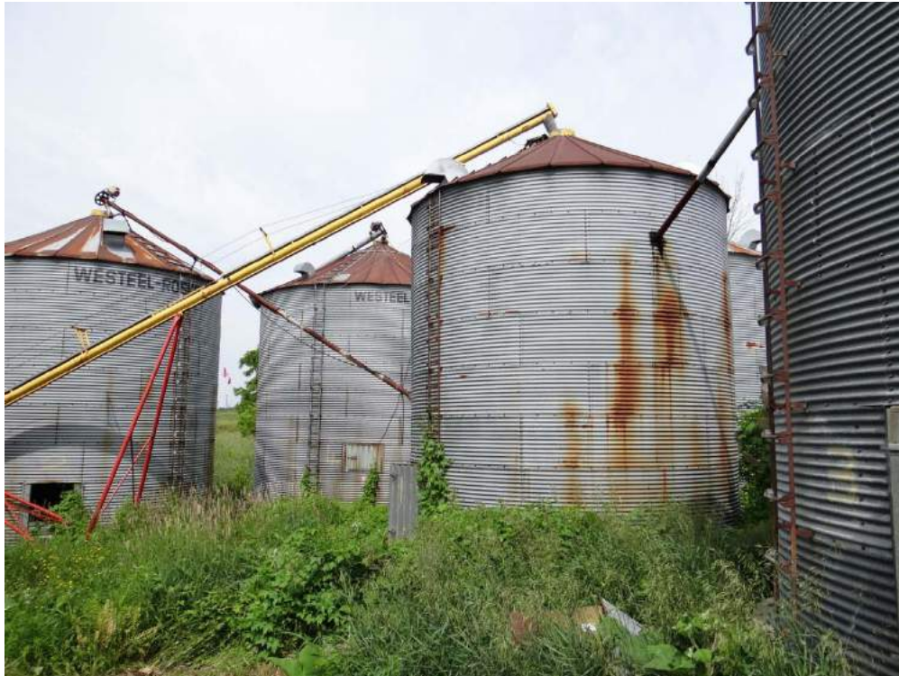
Plate 61: View towards the silos comprising the granary complex.
