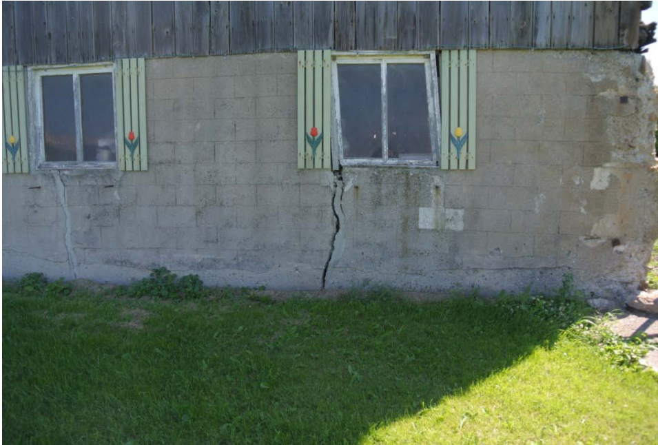
Plate 55: Detail of concrete foundations, west elevation. Note the incised lines in the concrete.
