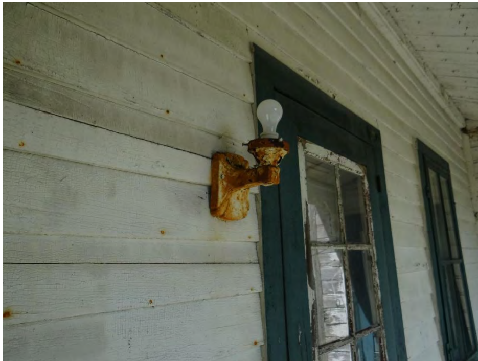
Plate 10: Photo showing clapboard siding on the east (front) elevation.
