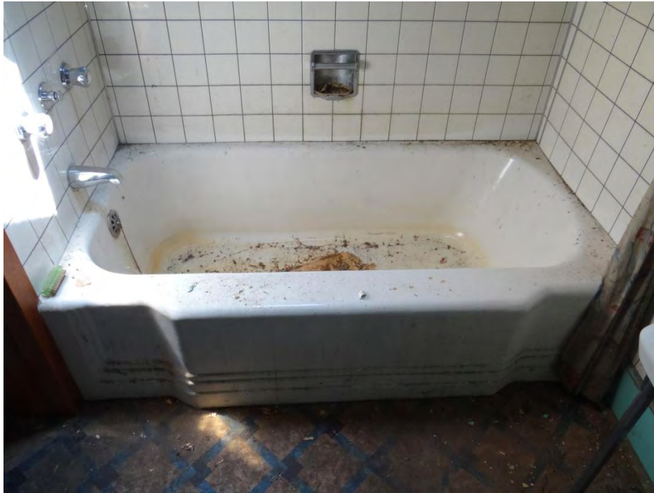
Plate 65: The bathtub in the second floor washroom.
