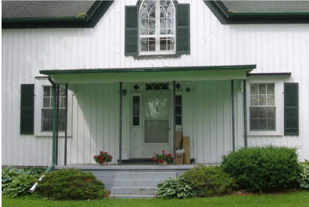
Plate 5: Detail of veranda on east elevation.
