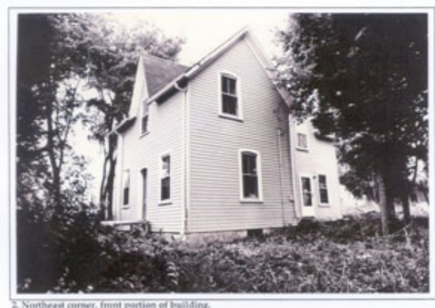
2. Northeast corner, front portion of building.
