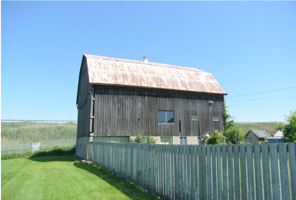
Plate 53: South and west elevations of the barn.
