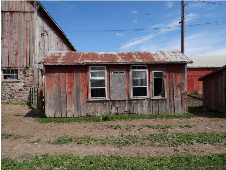
Plate 111: South elevation of outbuilding two (O2).
