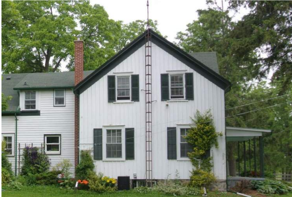
Plate 11: Detail of the south elevation of the original residence.
